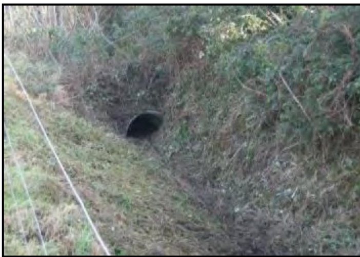
A ditch where silt has built up over the opening of an inlet pipe
