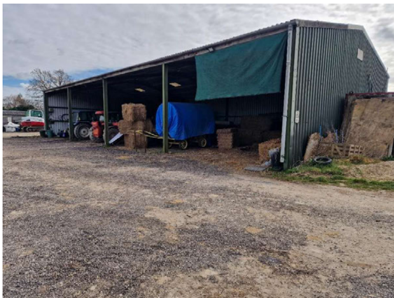
Photograph 2 North façade and access.
