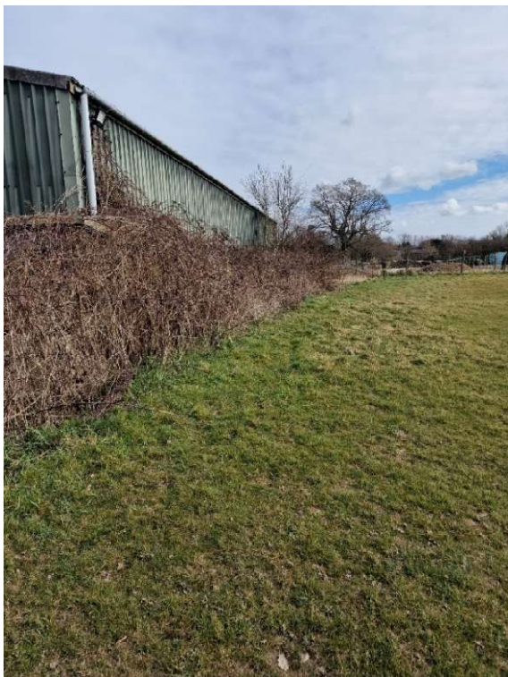
Photograph 1 Southern façade, adjacent to paddock
