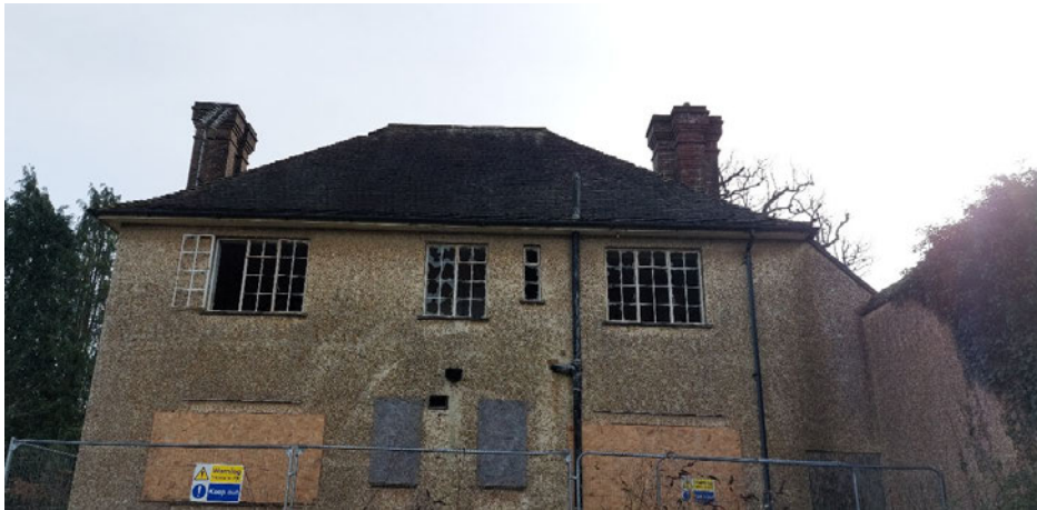
Image No. 04 – A view of the existing building.
