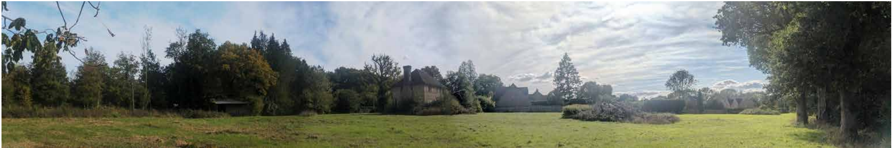
Photograph A. Southerly view of the eastern Site parcel, looking at the derelict house on Site, with the neighbouring property ( Pine Lodge ) behind. The tree lined eastern and northern boundaries are illustrated on the photograph. Brash piles within open grassland on sloping terrain provide the main Site characteristics.
