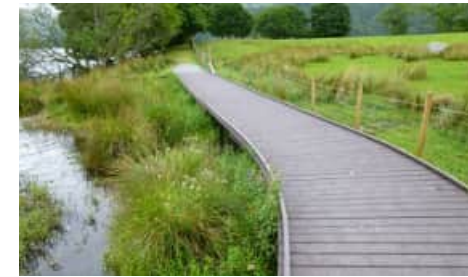
Pedestrian bridge crossing the stream
