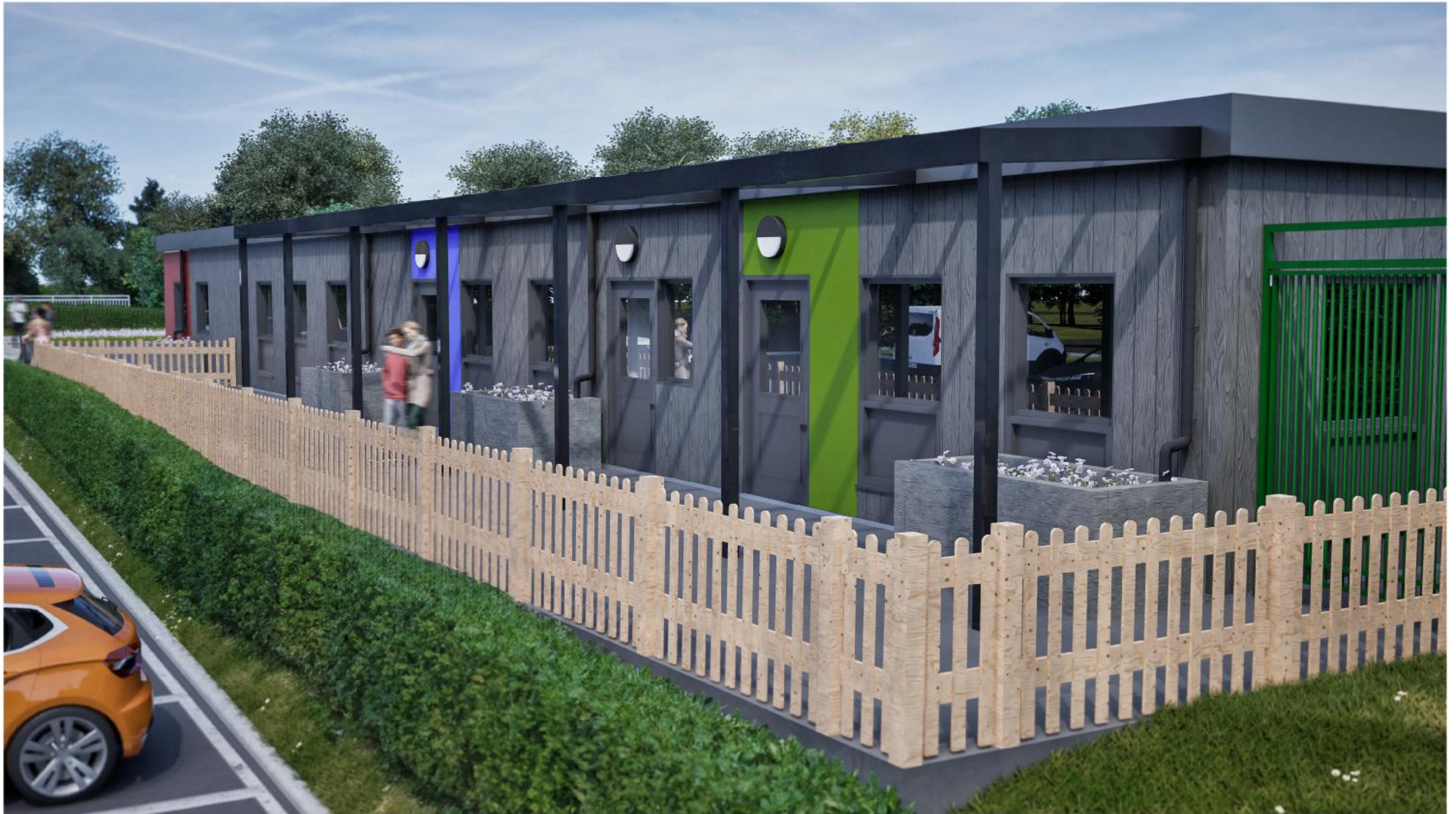
Phase 1 View of Northern Elevation
