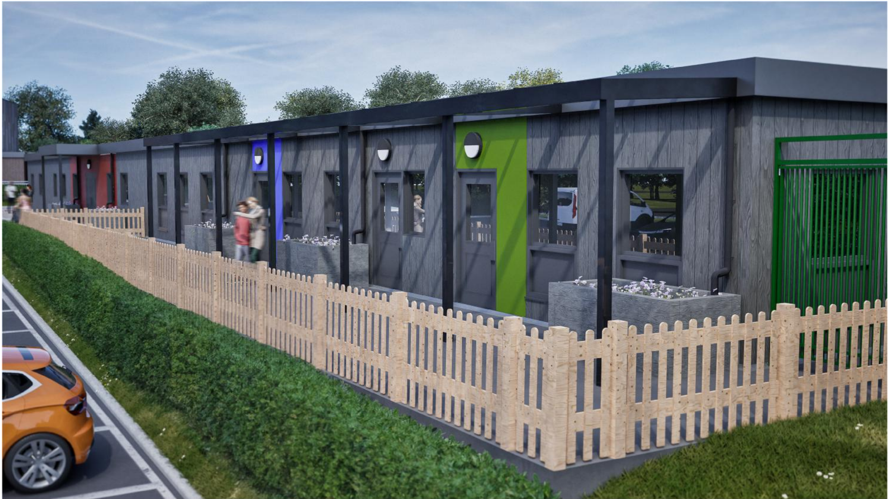
All Phases View of Northern Elevation
