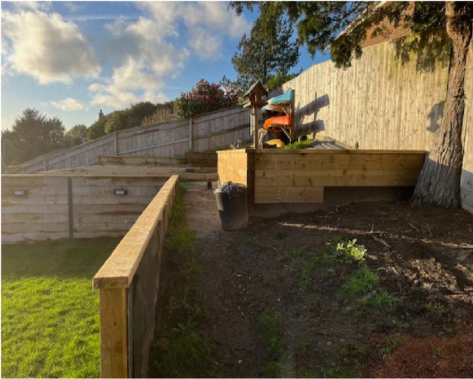
Photo 1 – Raised decking and walkway adjacent to the eastern boundary
