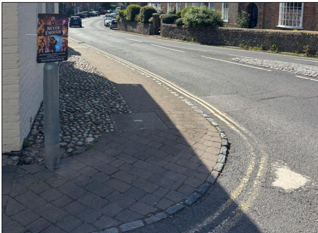
FIGURE 3-19: LACK OF PEDESTRIAN CROSSING OVER HIGH STREET MINI-ROUNDABOUT JUNCTION
