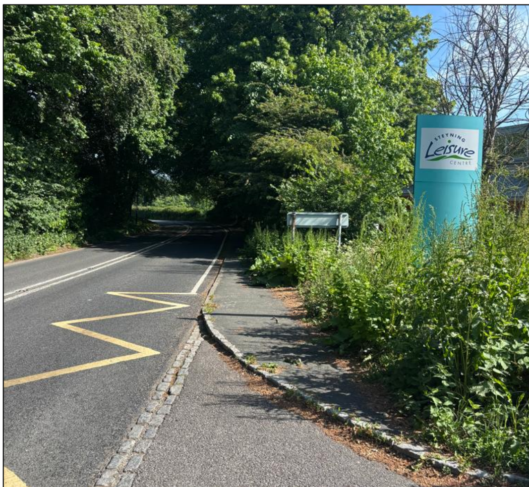
FIGURE 3-11: LACK OF DROPPED KERBS AND TACTILE PAVING AT LEISURE CENTRE ACCESS
