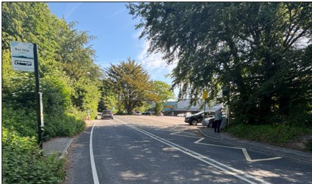
FIGURE 3-10: NORTHBOUND BUS STOP ON HORSHAM ROAD
