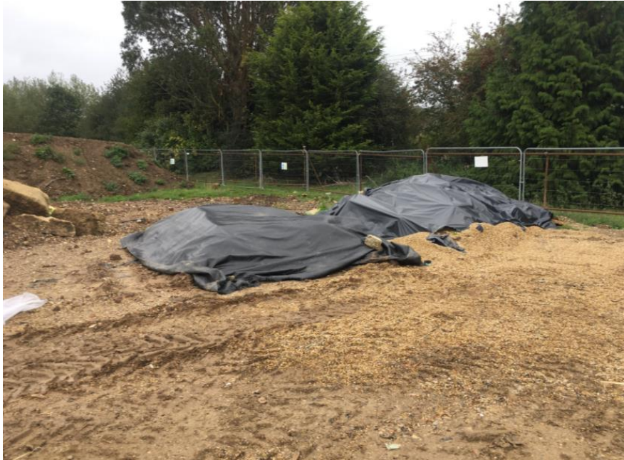
View of stockpiled soils for removal from site
