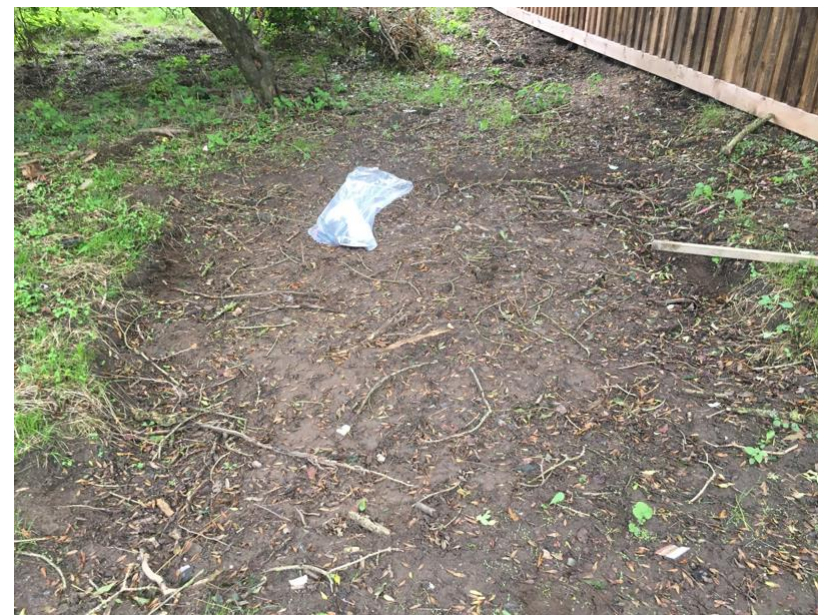
View of the 0.10m deep excavation
