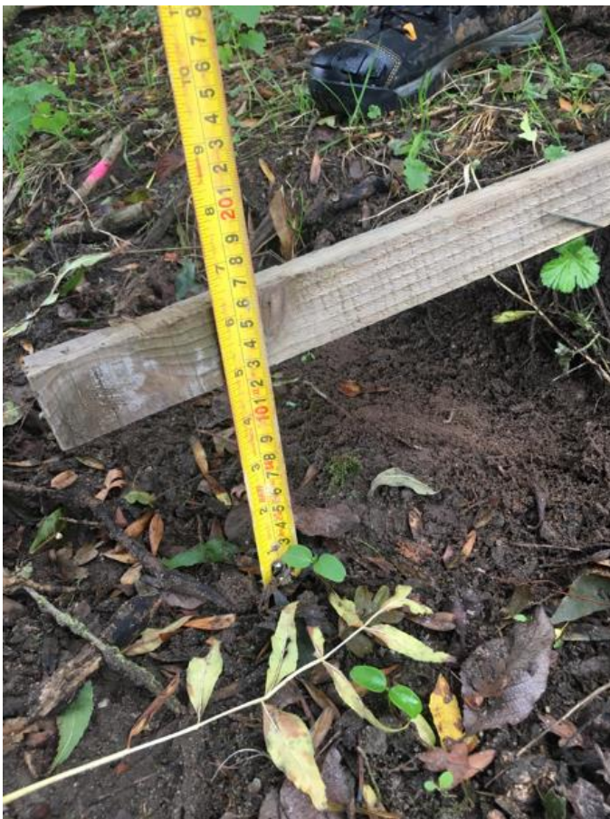
View of the 0.10m deep excavation – southern side
