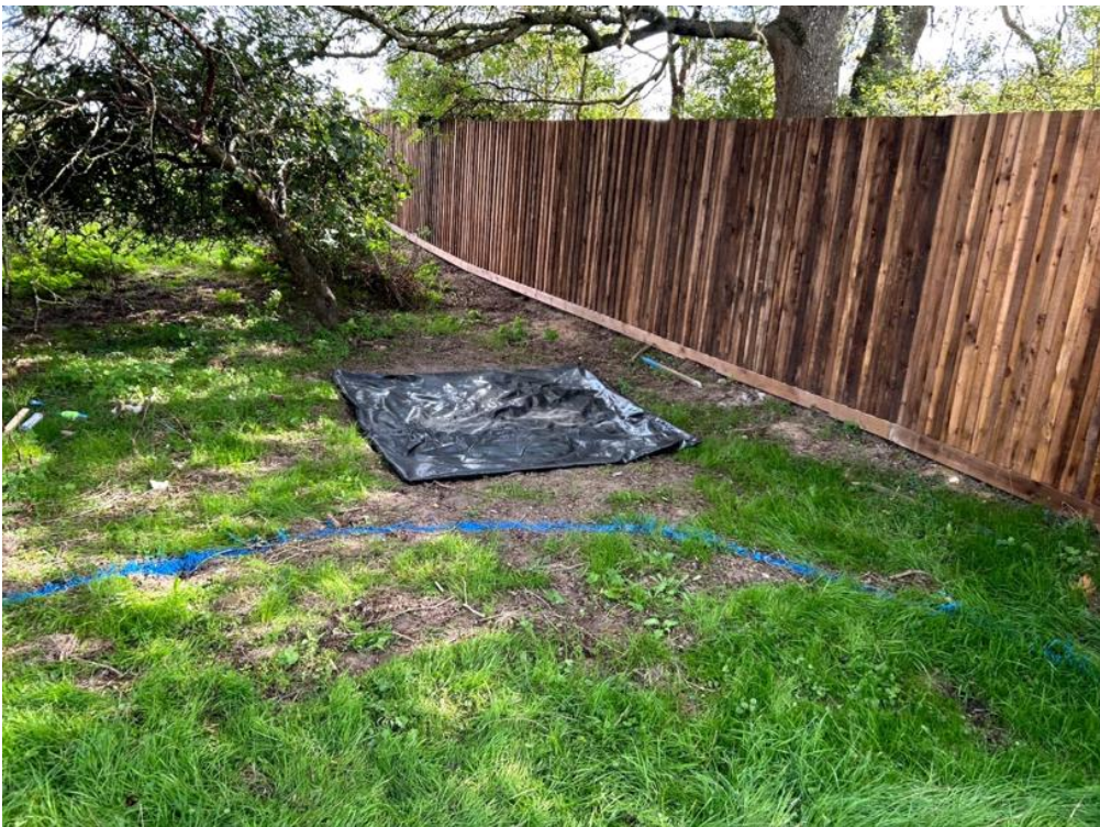
View of the membrane at the base of the excavation
