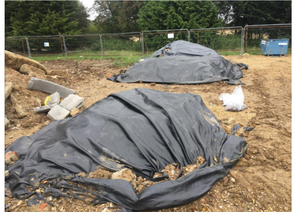
View of stockpiled soils for removal from site
