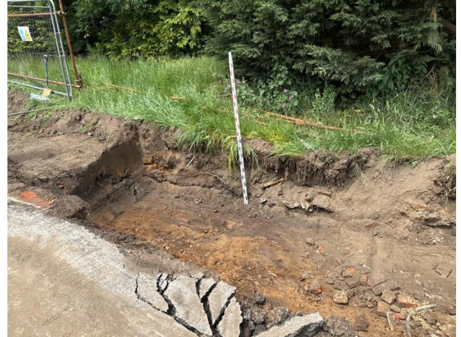
View of the 0.80m deep excavation
