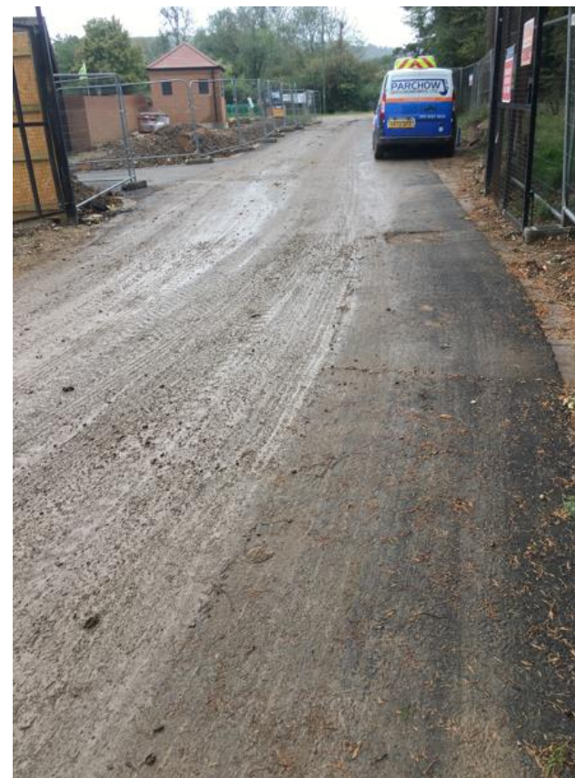
View of the completed access road covering the location of the former hot spot
