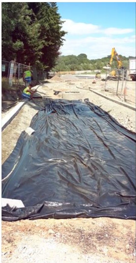
View of the membrane at base of the excavation
