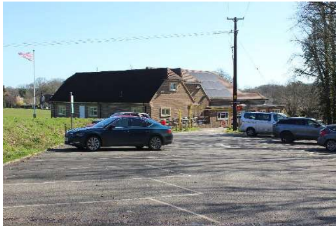
Image A - Barns Green Village Hall and car park to the north of the site
