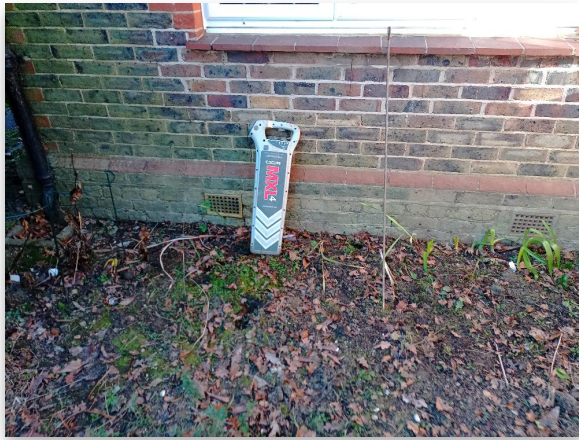
Fig 1.1: Trial Hole 1 Location
