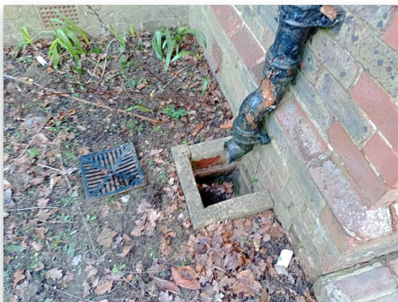
Fig 4.1: Rainwater Gully
