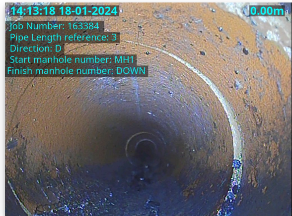
Fig 3.2: Line 3 Displacement
