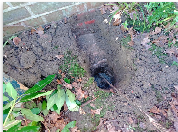
Fig 2.2: Trial Hole 2 Footing
