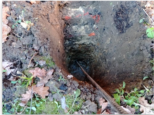
Fig 1.2: Trial Hole 1 Footing
