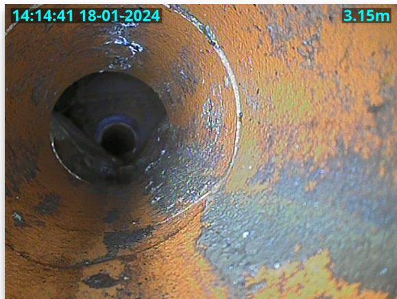
Fig 3.3: Line 1 Cracking
