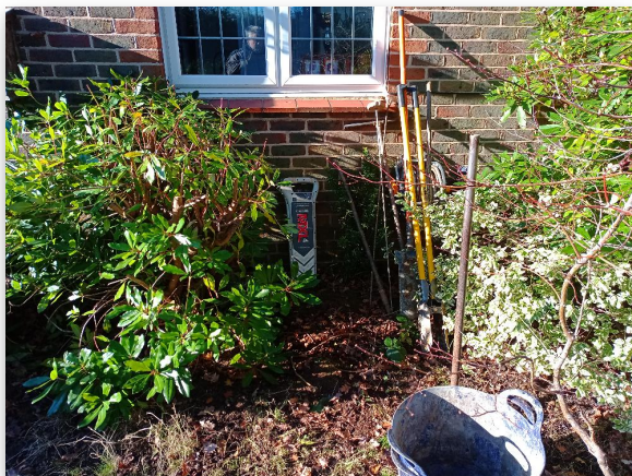
Fig 2.1: Trial Hole 2 Location
