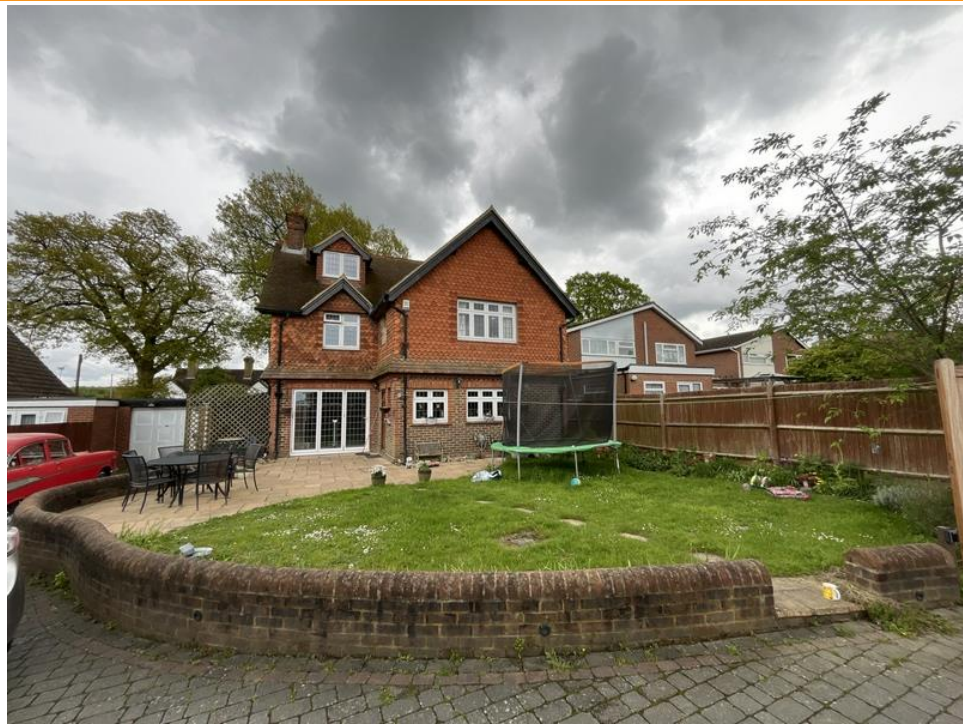
View of rear (lack of vegetation)
