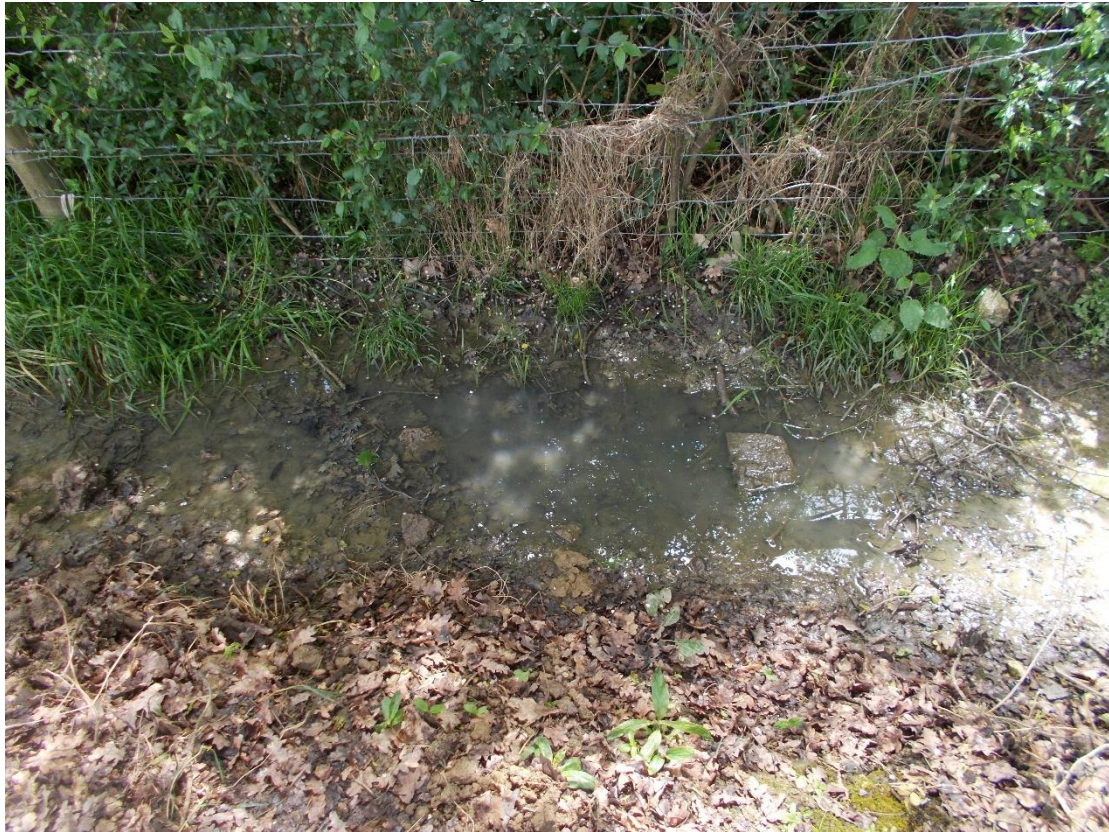
Drainage ditch south of site
