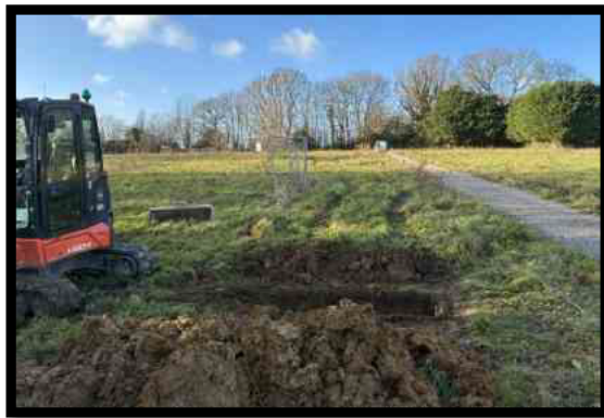
Trial pit 4 looking west
