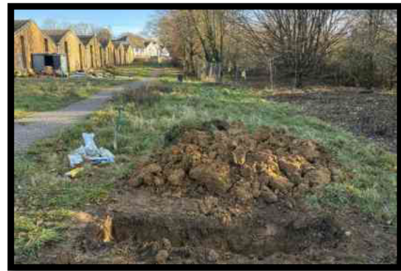
Trial pit 4 looking east
