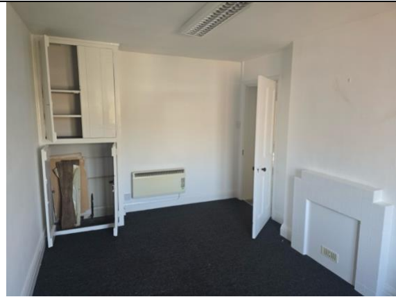
No 68 room F.04 (office)
