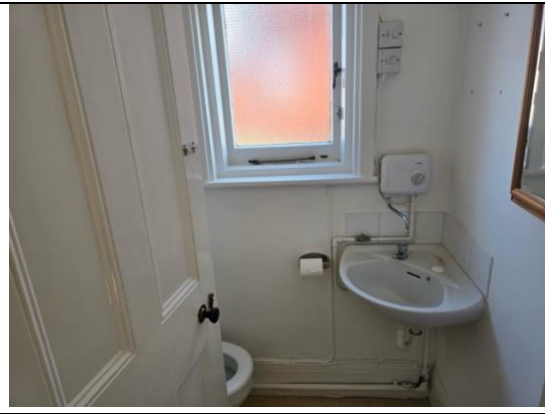
No 68 room G.03 (toilet)
