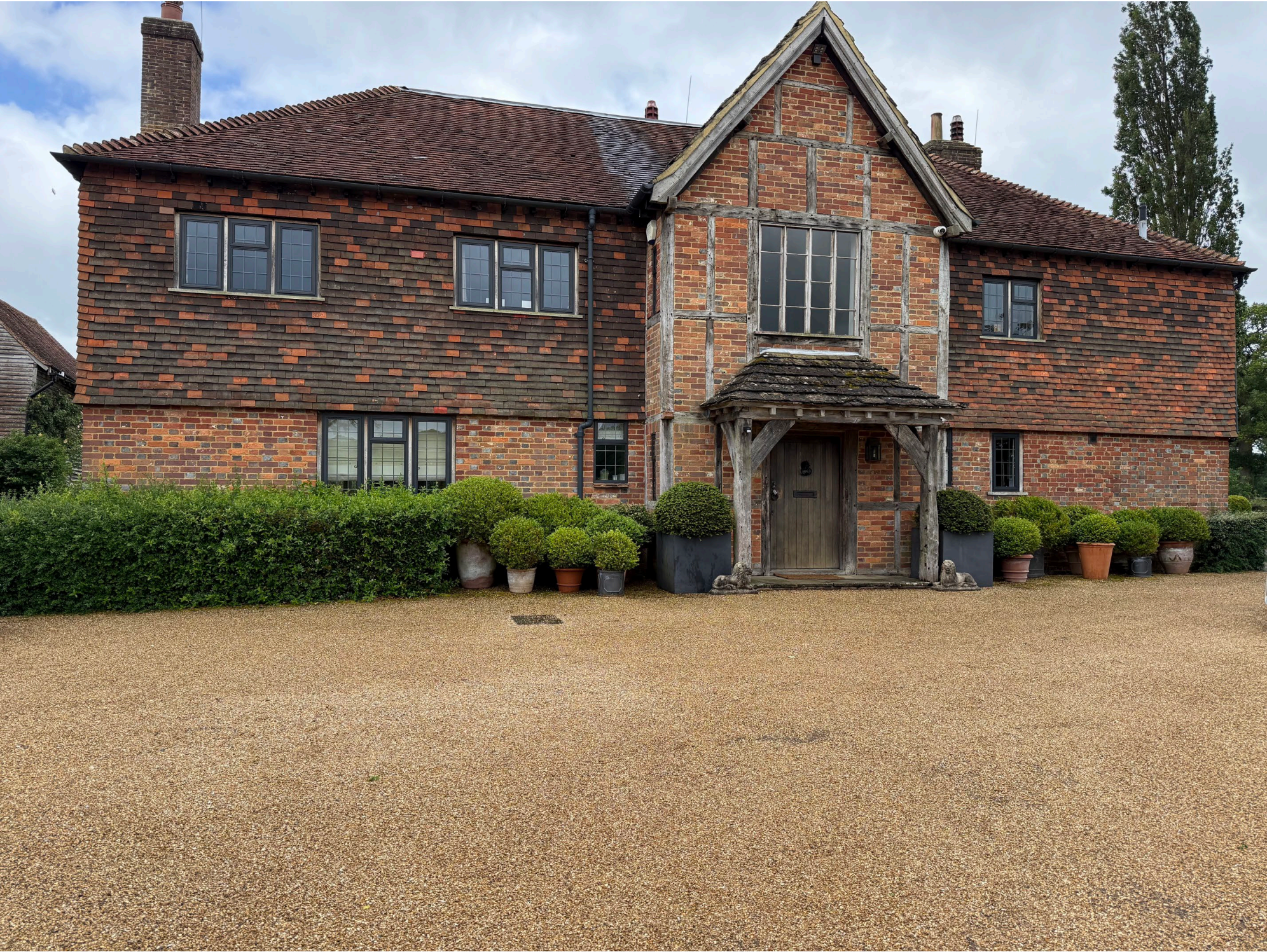
North Elevation (entrance)
