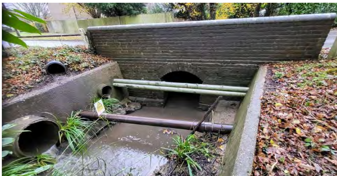
Photograph 1: Chapel Road Culvert (u/s)
