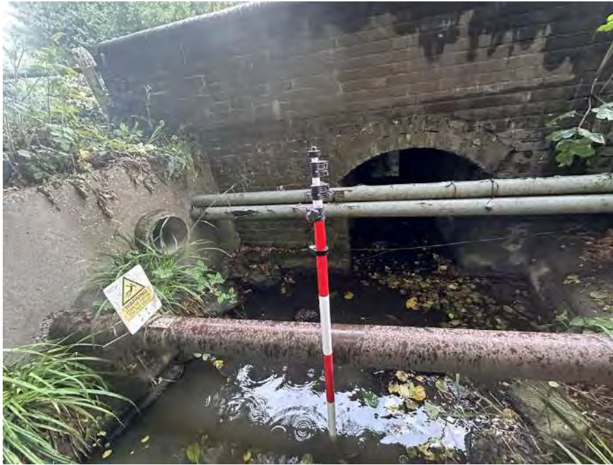
Fig.6 – Crossing pipe upstream of cross section MUNT01_00365.
