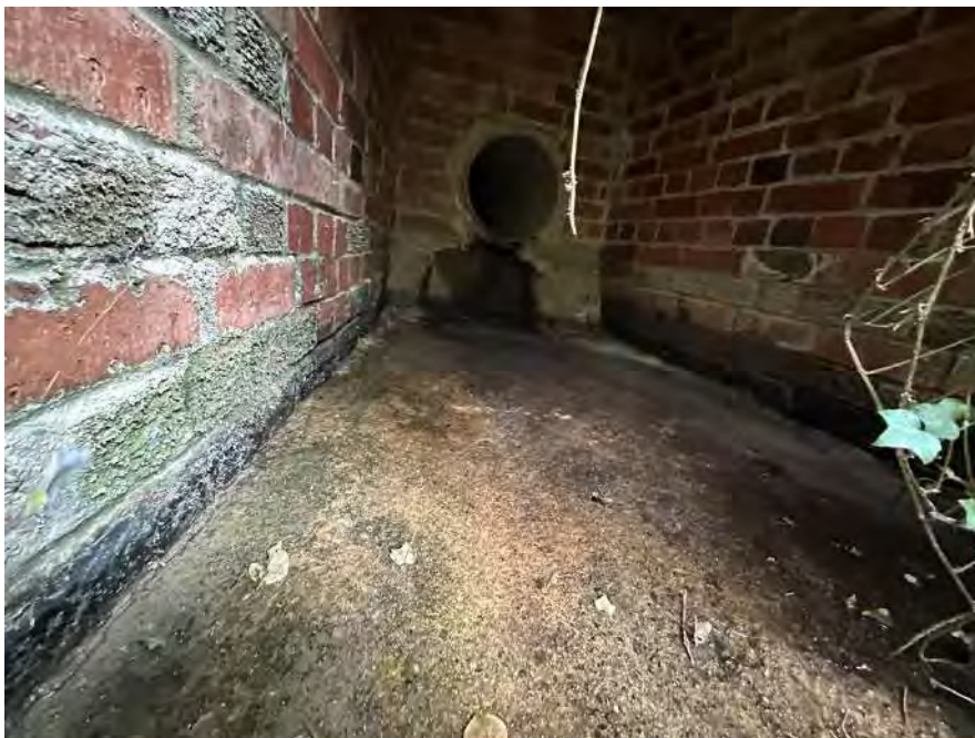
Fig.4 – Large left bank incoming pipe upstream of cross section MUNT01_00216.
