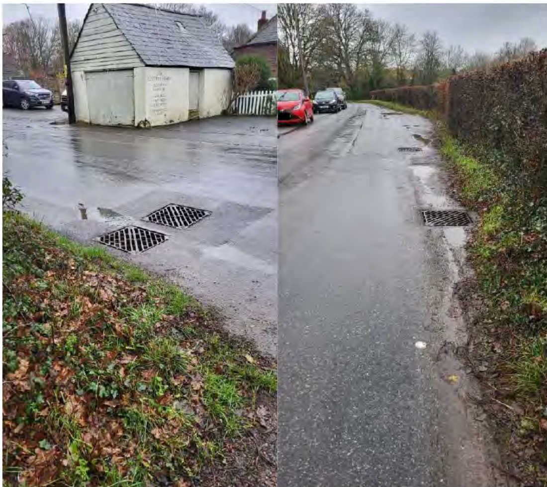
Photograph 2: Chapel Road Culvert Gullies
