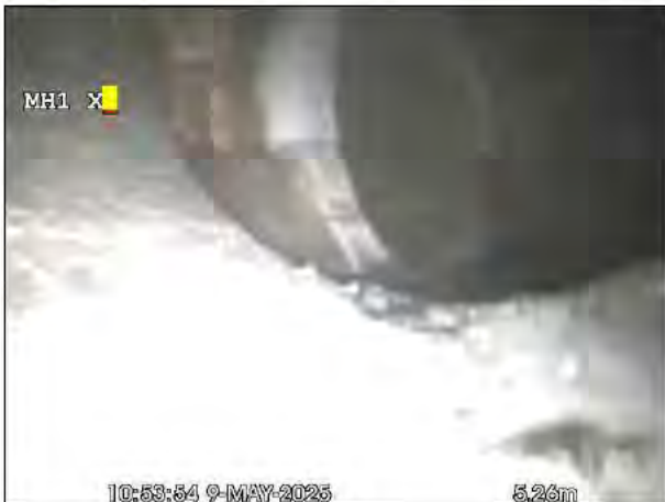
Photo: 36_8b, 00:00:00 5.5m, Finish Survey, Remark: MH visible
