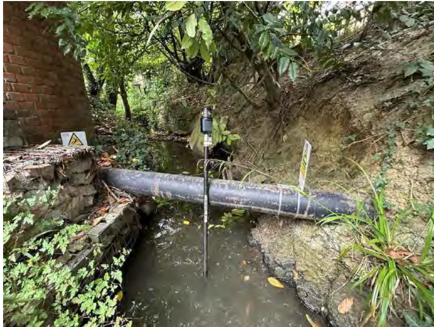
Fig.3 – Crossing pipe upstream of cross section MUNT01_00151.
