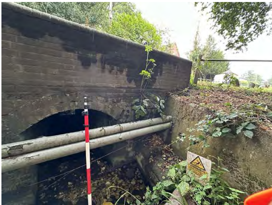
Fig.5 – Crossing pipe on structure face at cross section MUNT01_000365.
