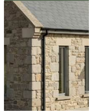
Stone Cornice and Quoin Detail
