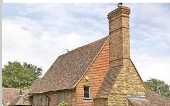
Gable and 'Sussex Stack' Chimney
