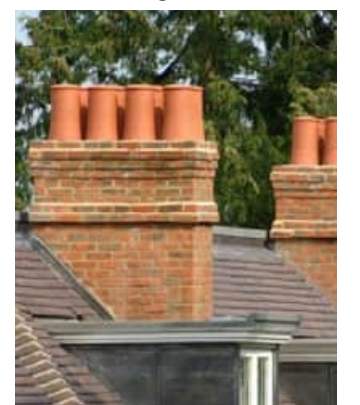
Sussex Stack Chimney
