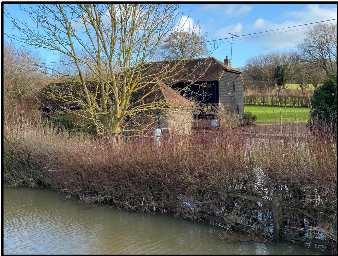
Photo 18: Little Barn (in Flood Zone 1) taken from the access track, approx. 300m south of the site. Dec. 2019
