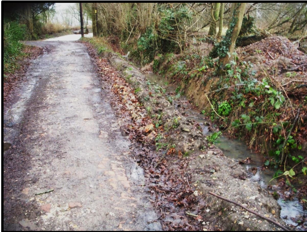
Photo 14: Hollands Lane in wet weather looking west towards the entrance to Rye House (which is on the left) with the drainage ditch along the north side of the lane taking runoff from the field.
