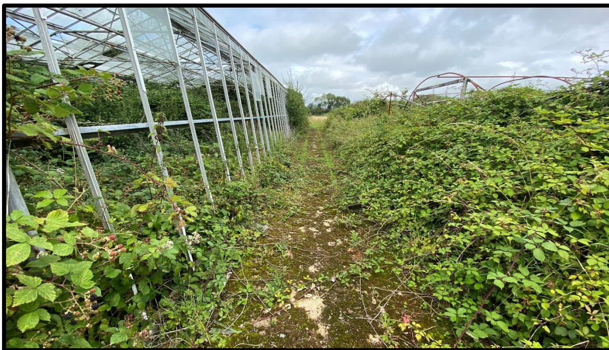
Photo 5: Concrete access track alongside the greenhouse looking north
