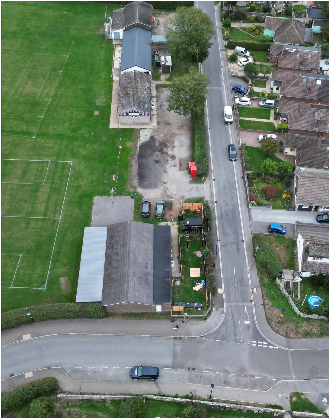
Figure 6 Church Lane Building Line
