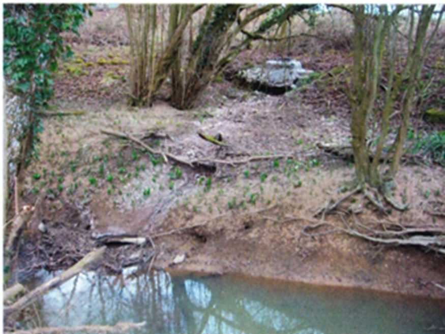
View of the Incoming Sewer Manhole Located Just Upstream of the Raw Sewage Lift Pumping Station in the Treatment Plant with Parsons Brook in the Foreground
