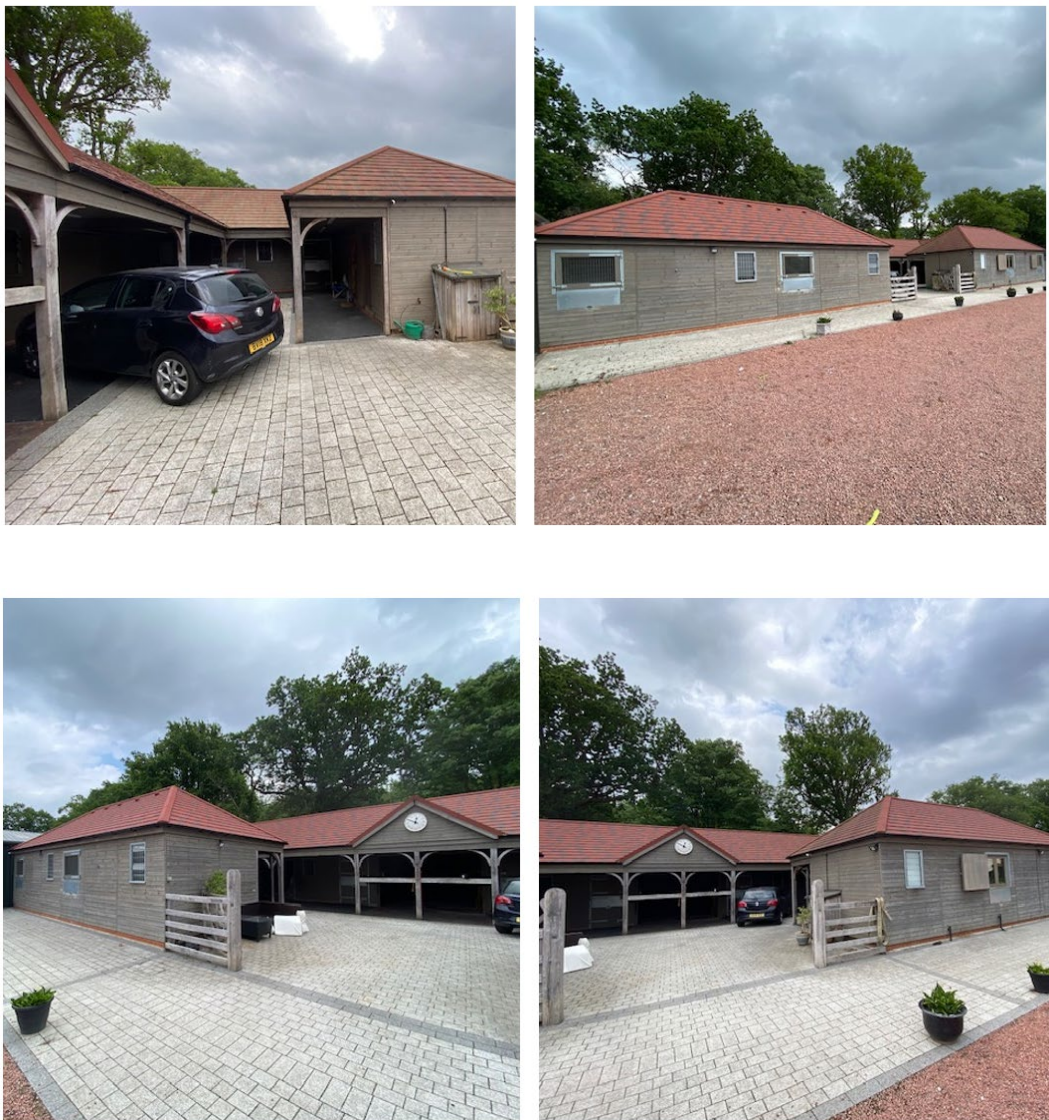
Figure 2.2 – Site photographs of existing stables and hard standing
