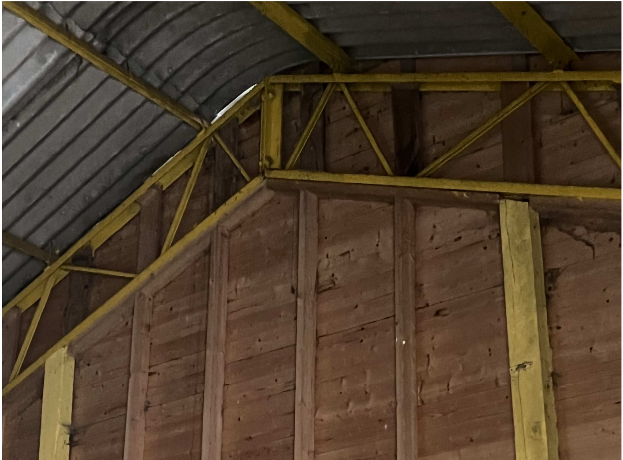
Gable end – truss rafters and posts. Vertically spanning timbers.
