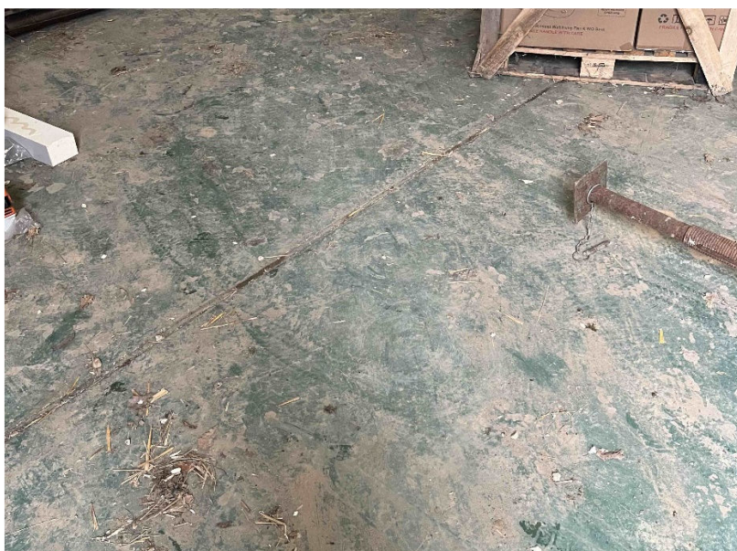
Floor was in good condition.
