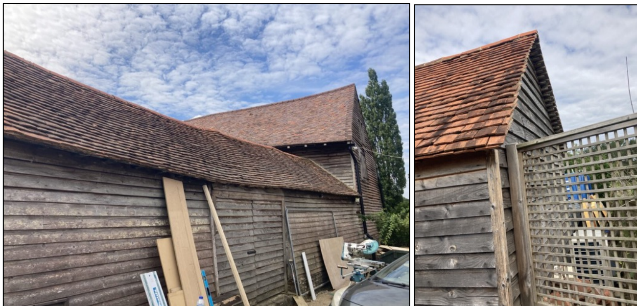
Photograph 5a & 5b. The northern pitch (left) and eastern gable (right) of the covered walkway at Town House Farm.
