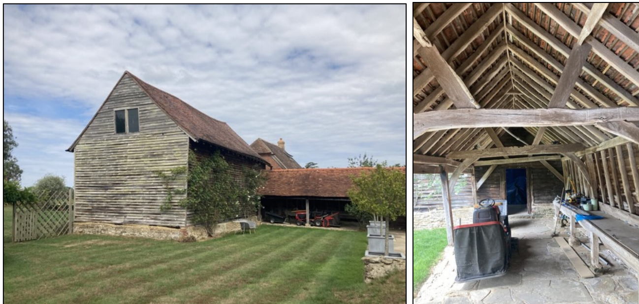
Photograph 3a & 3b. The southern and eastern elevations of the barn (left) where the covered walkway attaches, with a view of the open section within this walkway (right).
