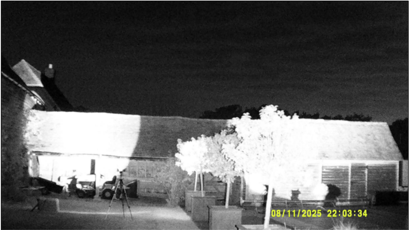
Figure 3. Darkest point of the night vision camera covering the southern pitch of the covered walkway on the barn at Town House Farm during the survey on 11 th August 2025.
