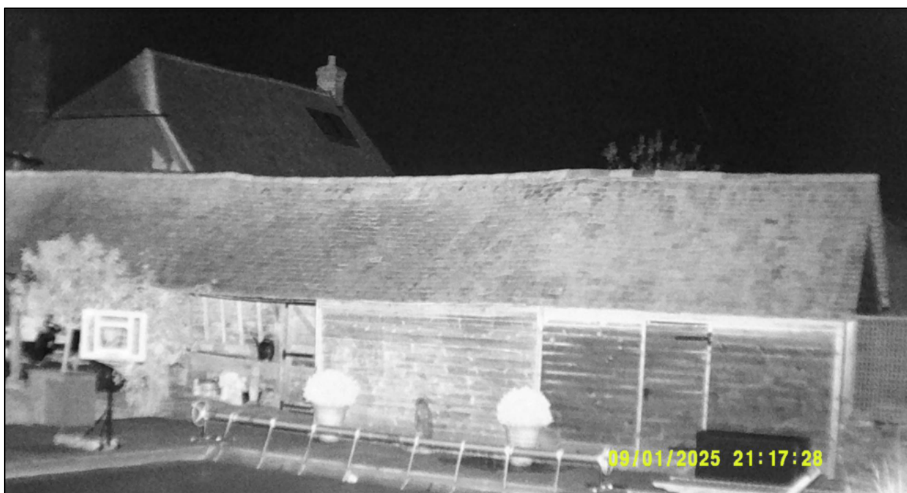
Figure 8. Darkest point of the night vision camera covering the eastern section and eastern gable end of the southern pitch of the covered walkway on the barn at Town House Farm during the survey on 1 st September 2025.
