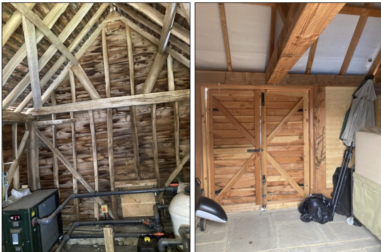
Photograph 4. Interiors of the two store sheds within the covered walkway, including the original shed housing the air conditioning unit (left), and the newer build used for storage (right).
