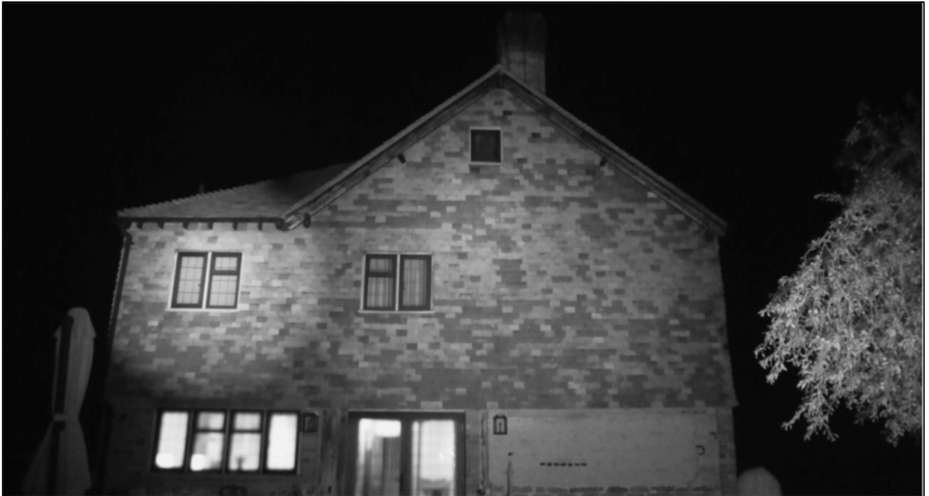
Figure 5. Darkest point of the night vision camera covering the western elevation of the house at Town House Farm during the survey on 1 st September 2025.
