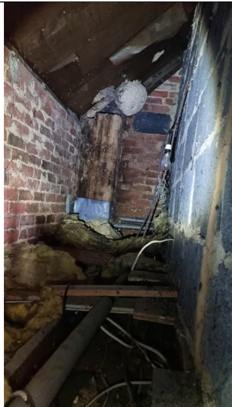
Plate 11. Dwelling crawl space
