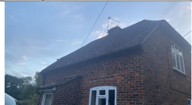
Figure 6: Eastern elevation of B1
