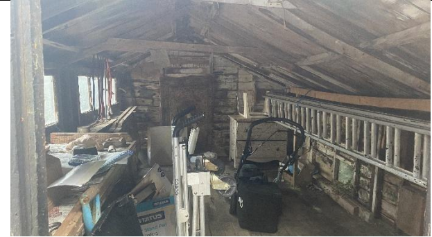
Figure 8: Interior of B2
