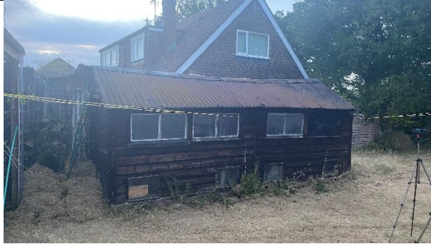
Figure 7: Exterior of B2
