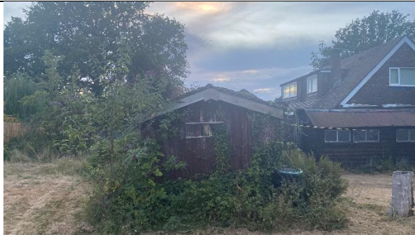
Figure 9: Exterior of B3
