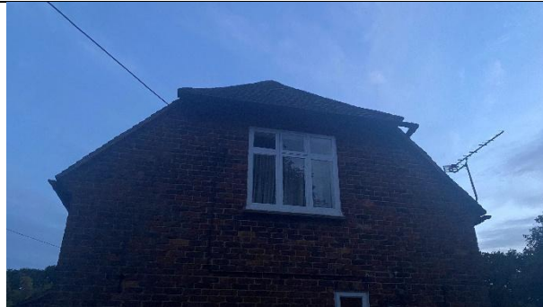
Figure 5: Northern elevation of B1
