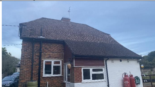
Figure 7: Western elevation of B1
