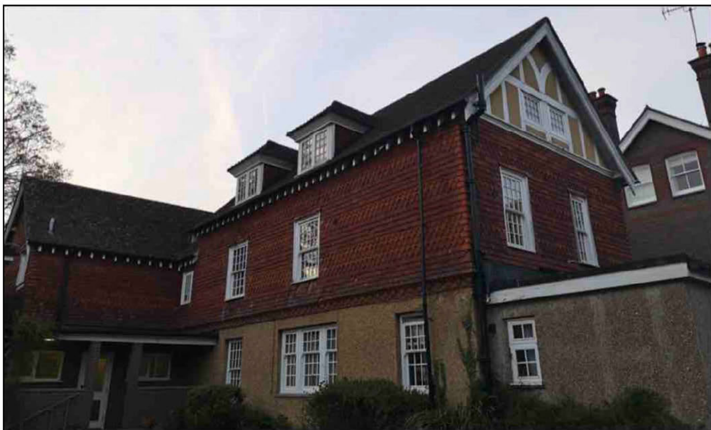
Example of a residential dwelling in Handcross, similar in style and status as The Warren.
