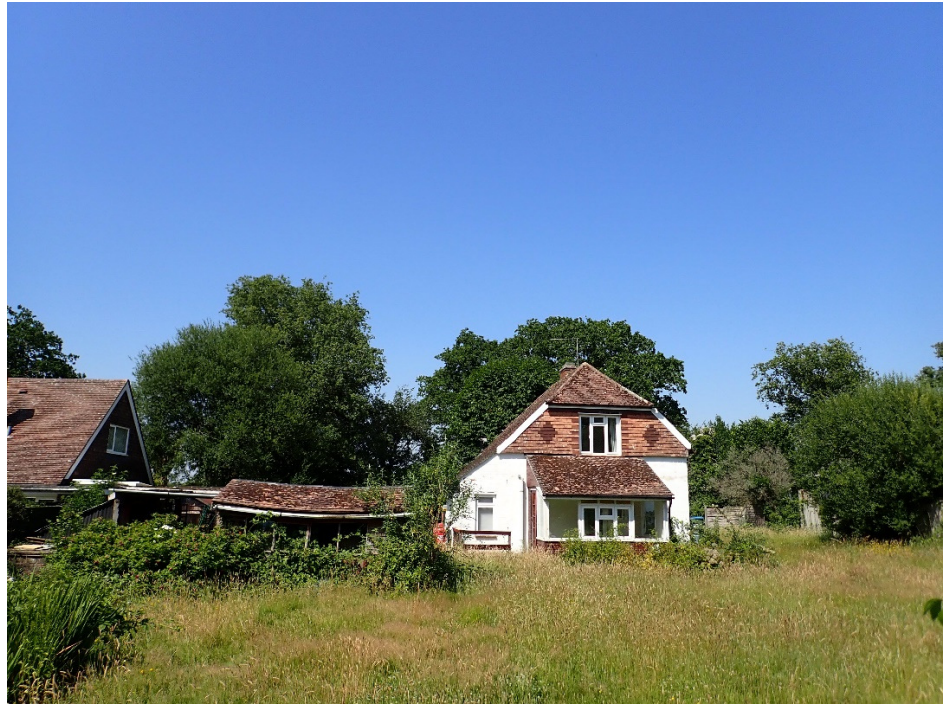
2.3 Rear of existing property, viewed from the South
