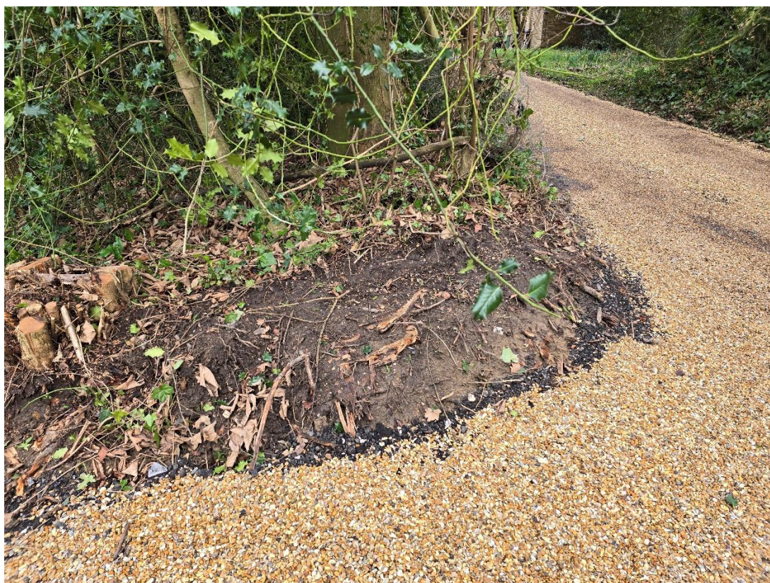
Photo 2 – Historic root damage at the base of T002 (Sycamore)
