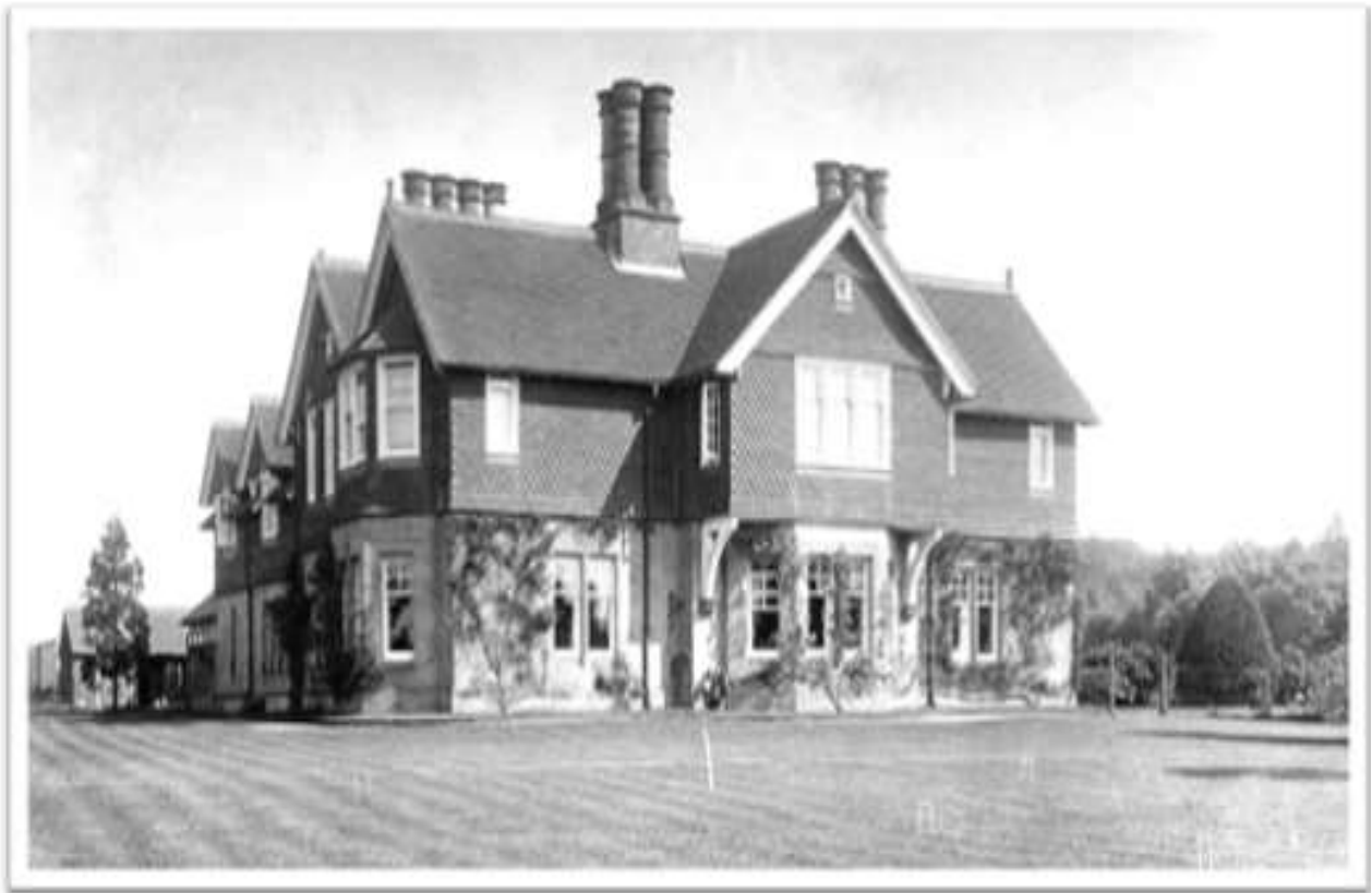
The Warren mansion and outbuildings, 1908. Source: Slaugham Archives
