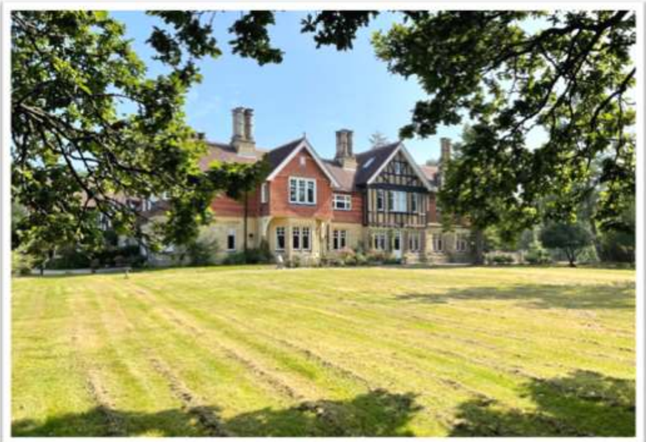
The mansion was extended 1910-12 and converted to 11 flats in 1965 (photo 2020)
