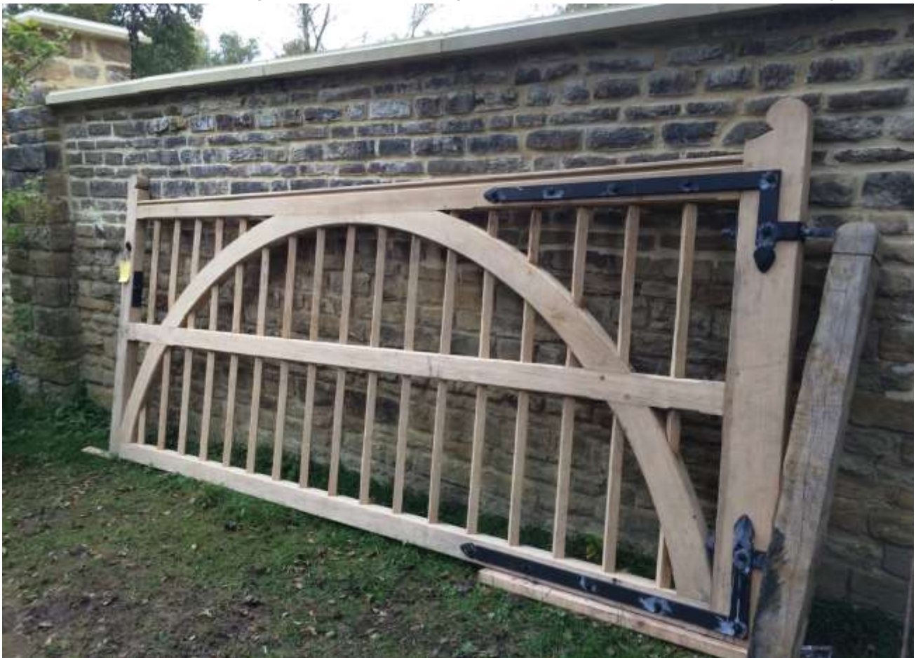
Restoration of walls and gates at Warren Virgate to Back Drive and the memorial garden
