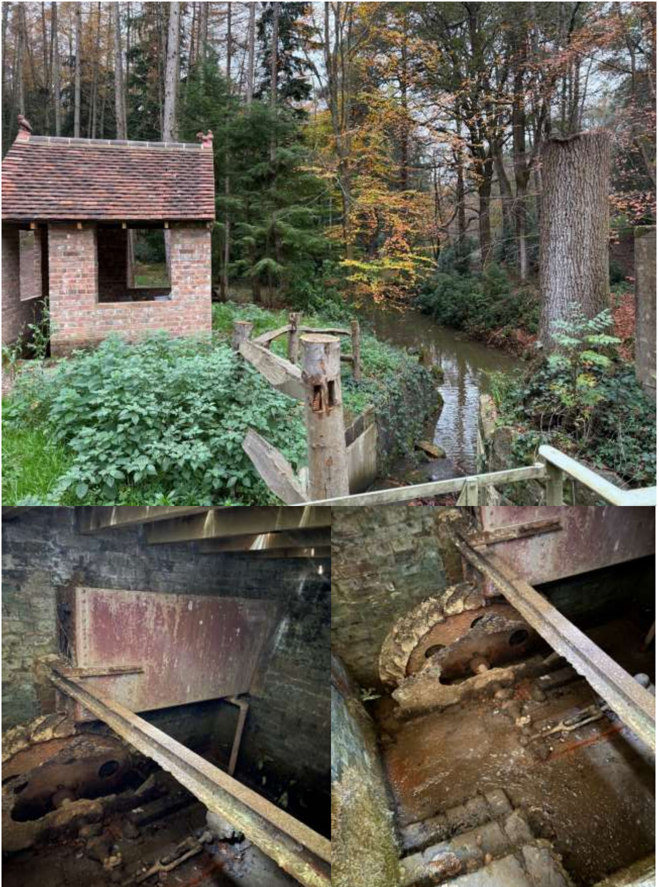
Restoration has begun on the 19 th century pump house and electric generator
