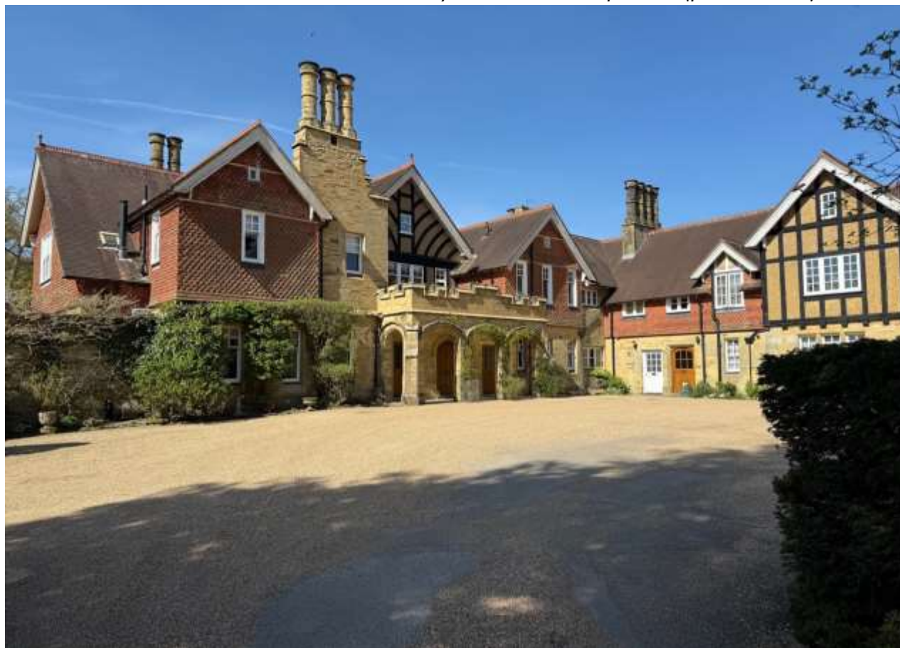
Restored sash windows, materials, chimneys and entrance portico (photo 2025)
