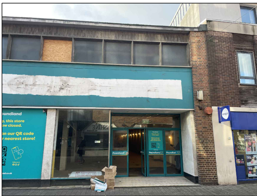
Photograph #2 (Dec '25) Existing Front Elevation - RHS
