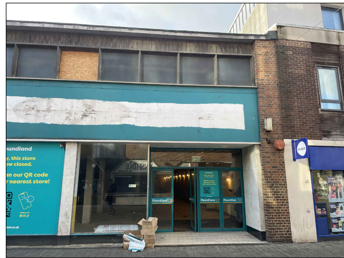
Photograph #2 (Dec '25) Existing Front Elevation - RHS
