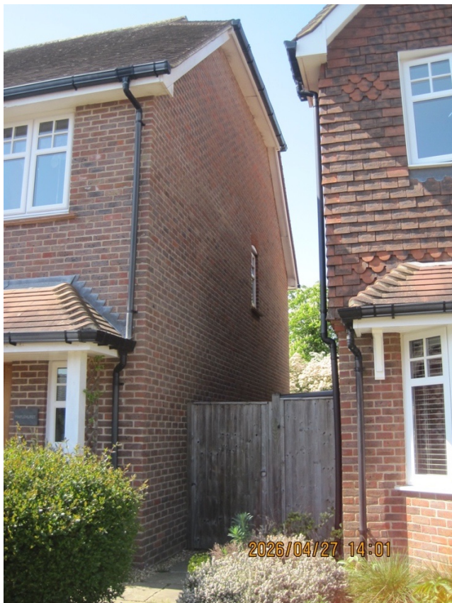
Maplehurst side (from front) showing first floor landing window
