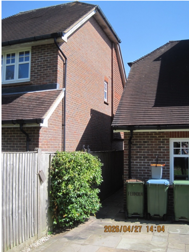
Westwood side facing Fernden (from rear) showing first floor obscure glazed bathroom window
