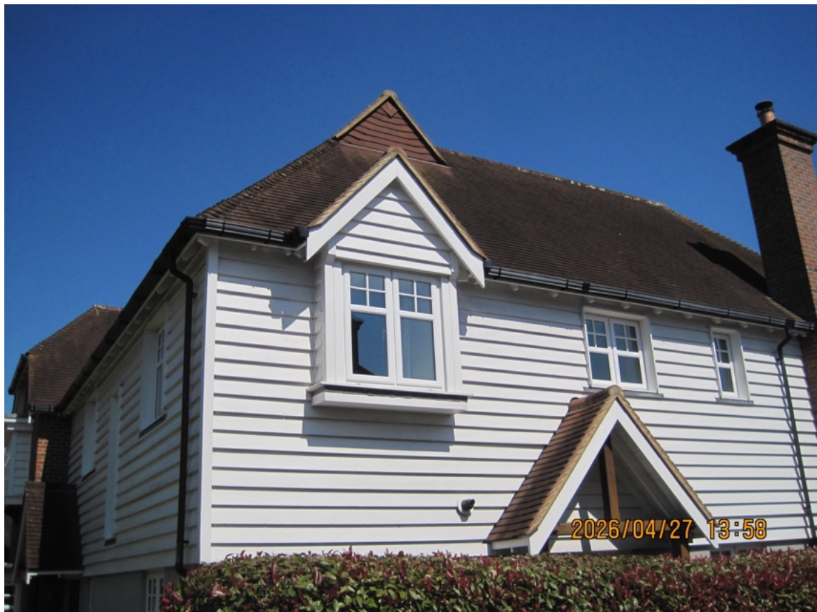
Nearby Amberley House showing example of first floor box bay
