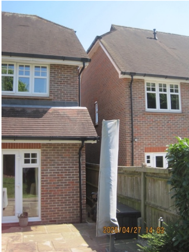
Maplehurst side (from rear) showing first floor landing window
