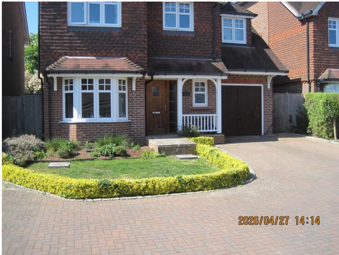
Fernden front showing area for new parking space adjacent existing spaces
