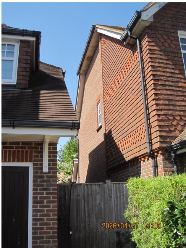
Westwood side facing Fernden (from front) showing first floor obscure glazed bathroom window
