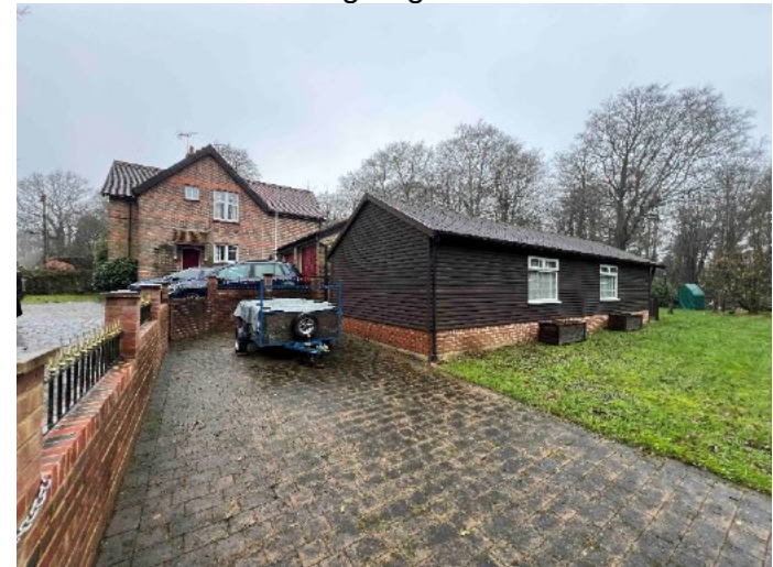
Rear and east elevation of annex
