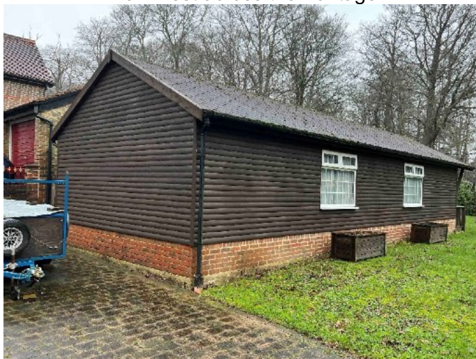
Rear and east elevation of annex
