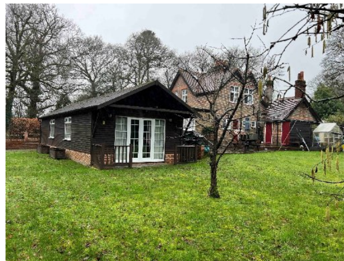
Front (north) elevation of annex from garden
