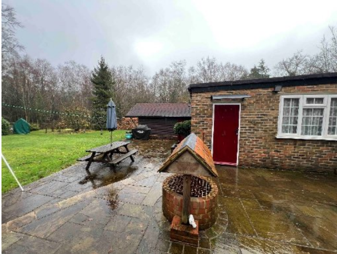
West elevations of garage and annex
