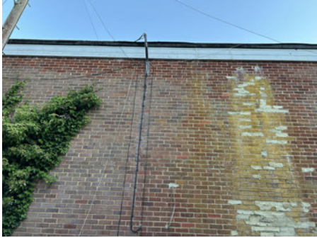
Concrete infill in brick work on northeastern elevation of B1.
