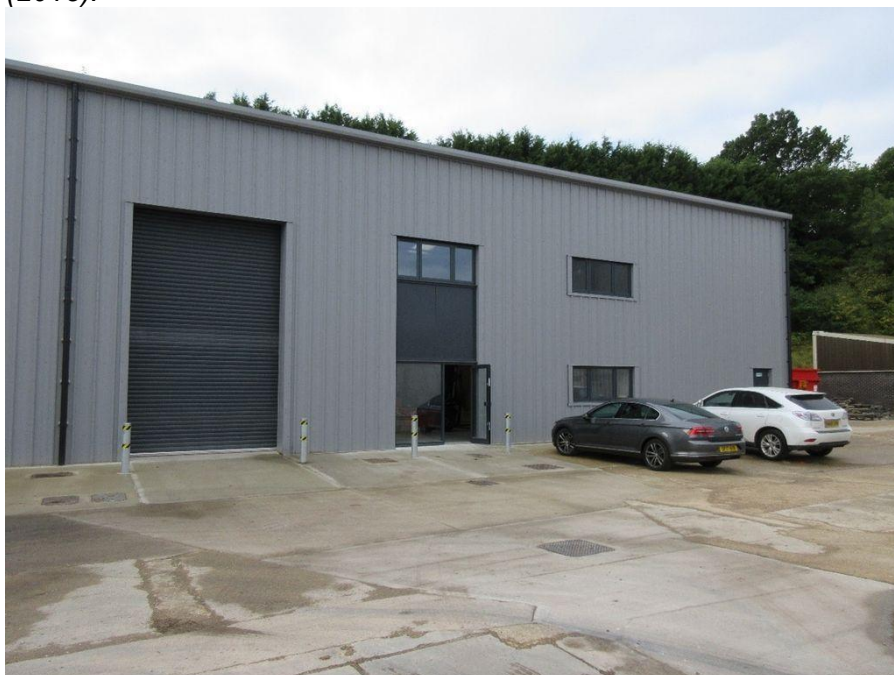
Building 3 - West Unit
