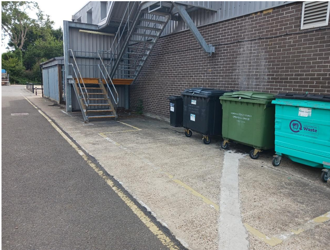
Building 3 – East Flank
