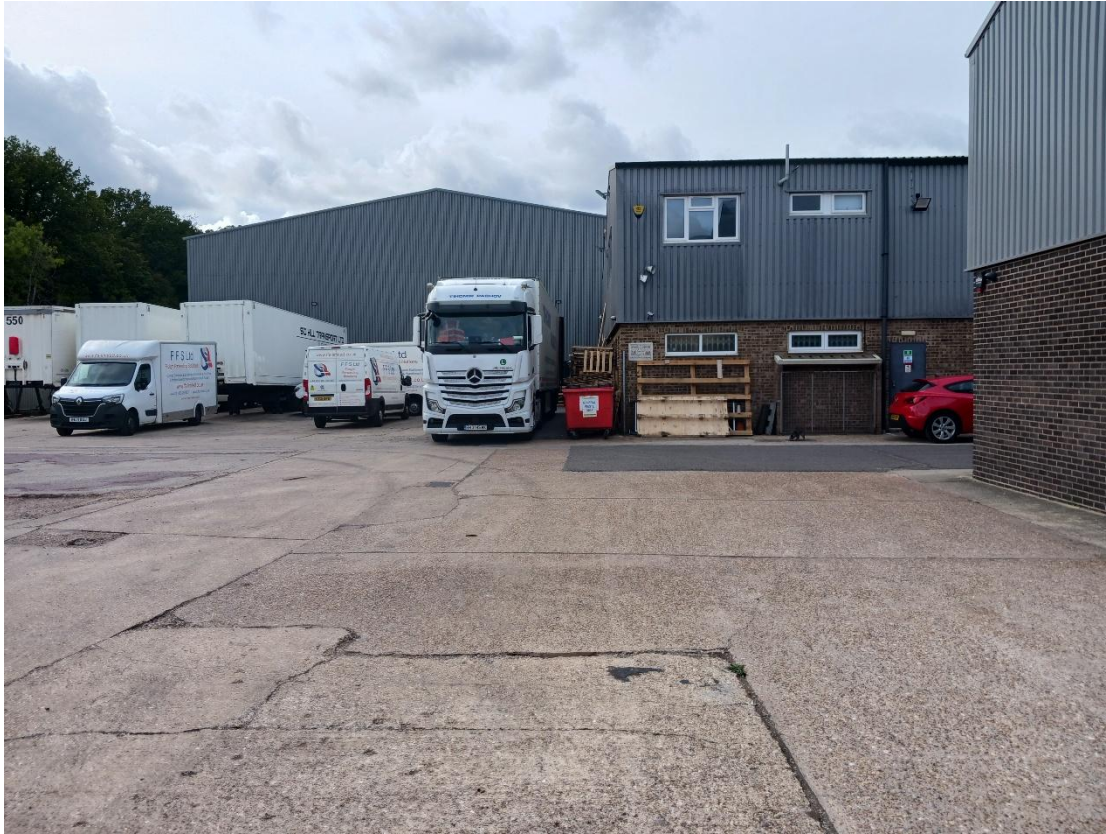
Building 2 – Rear Corner
