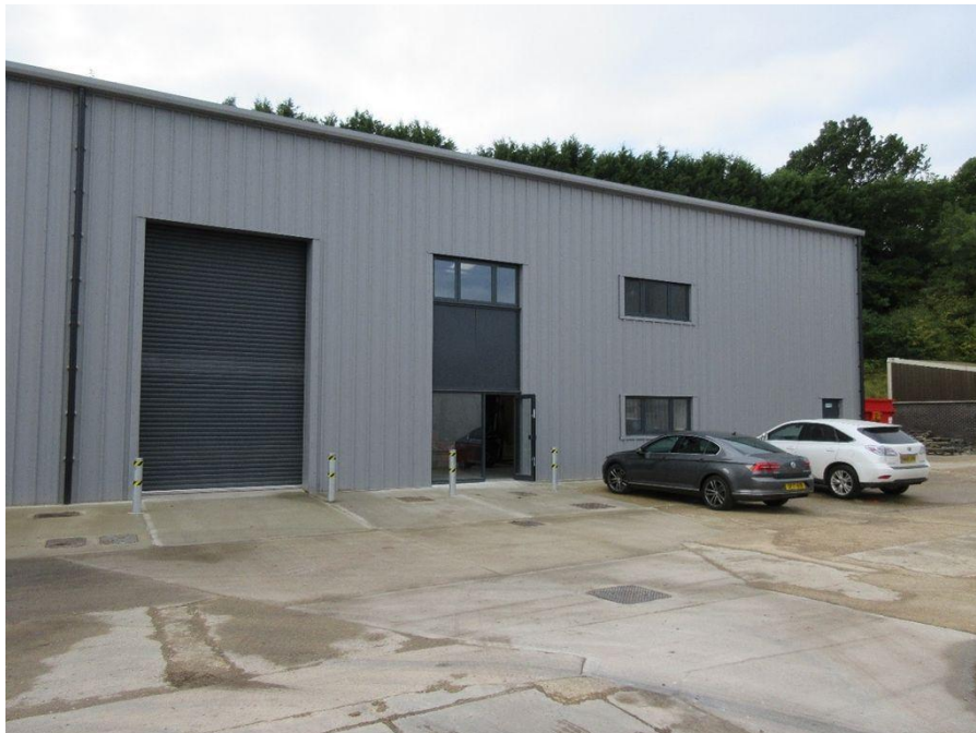
Building 3 - West Unit
