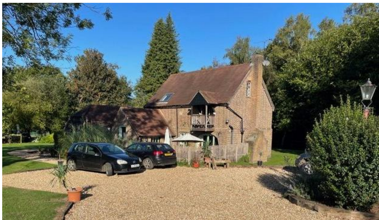
South and East Elevations
