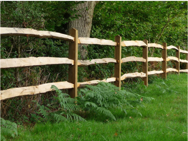
TIMBER POST AND RAIL CLEFT FENCE
