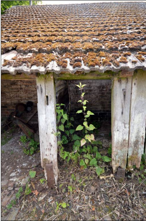
Plate 13: The southern doorway in the west wall of the yard with a view into the yard towards the stalls
