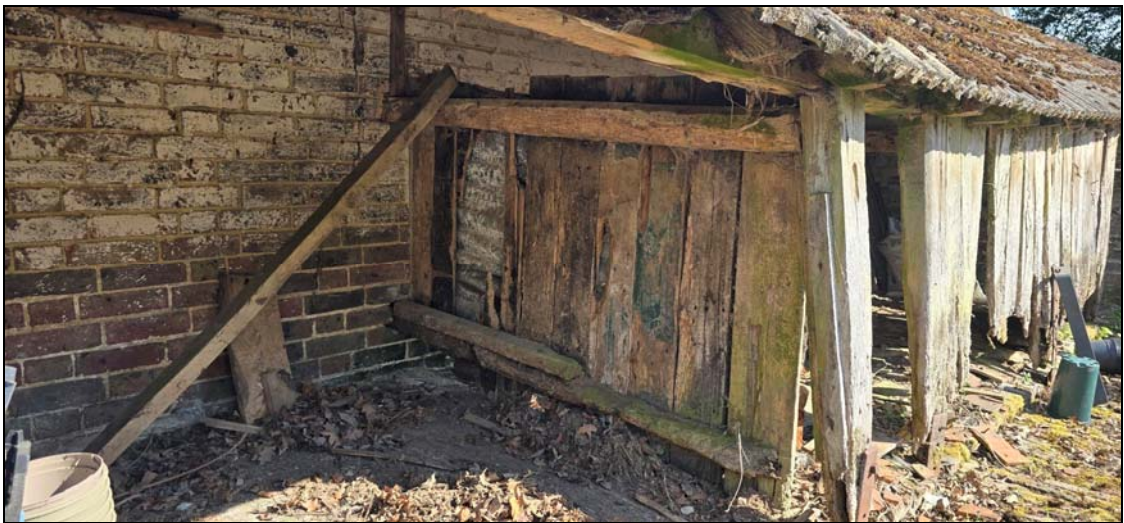
Plate 9: Light-weight partitioning between the stalls in the lean-to outshot (image provided by the owner)
