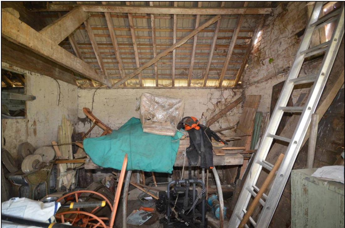
Plate 16: The east slope of the south room with its nailed-on diagonal brace
