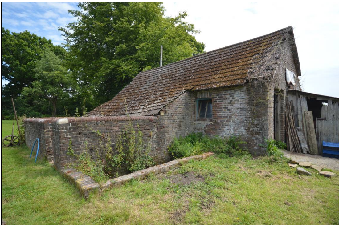
Plate 7: The group showing the brickwork of the external elevations, including the lining of the slurry pit
