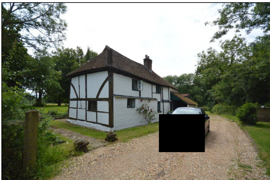
Plate 17: The north and west elevations of the domestic dwelling at Harwoods
