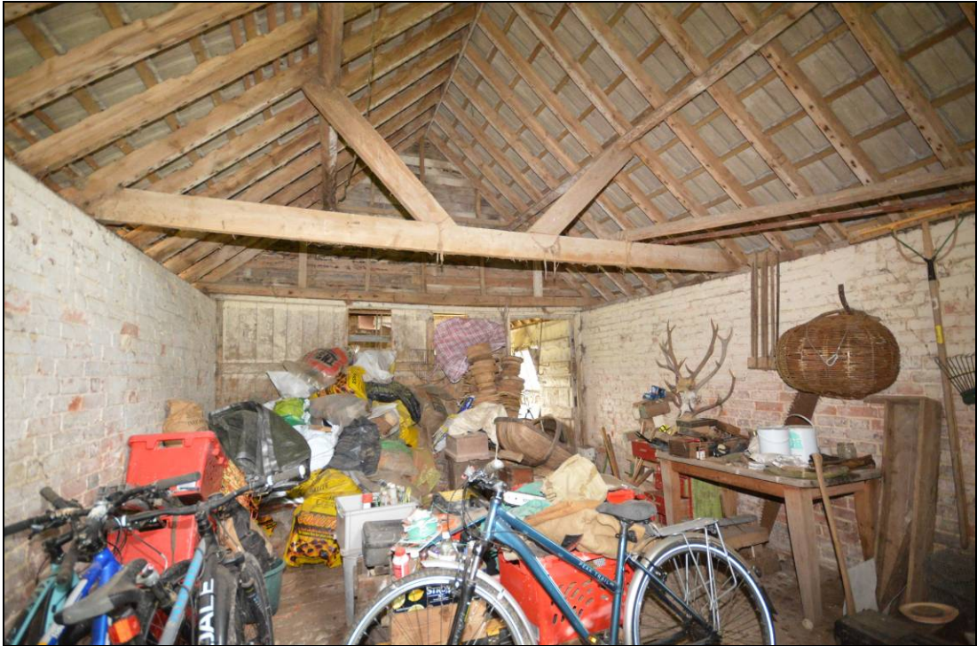
Plate 15: The interior of the north room showing the roof construction
