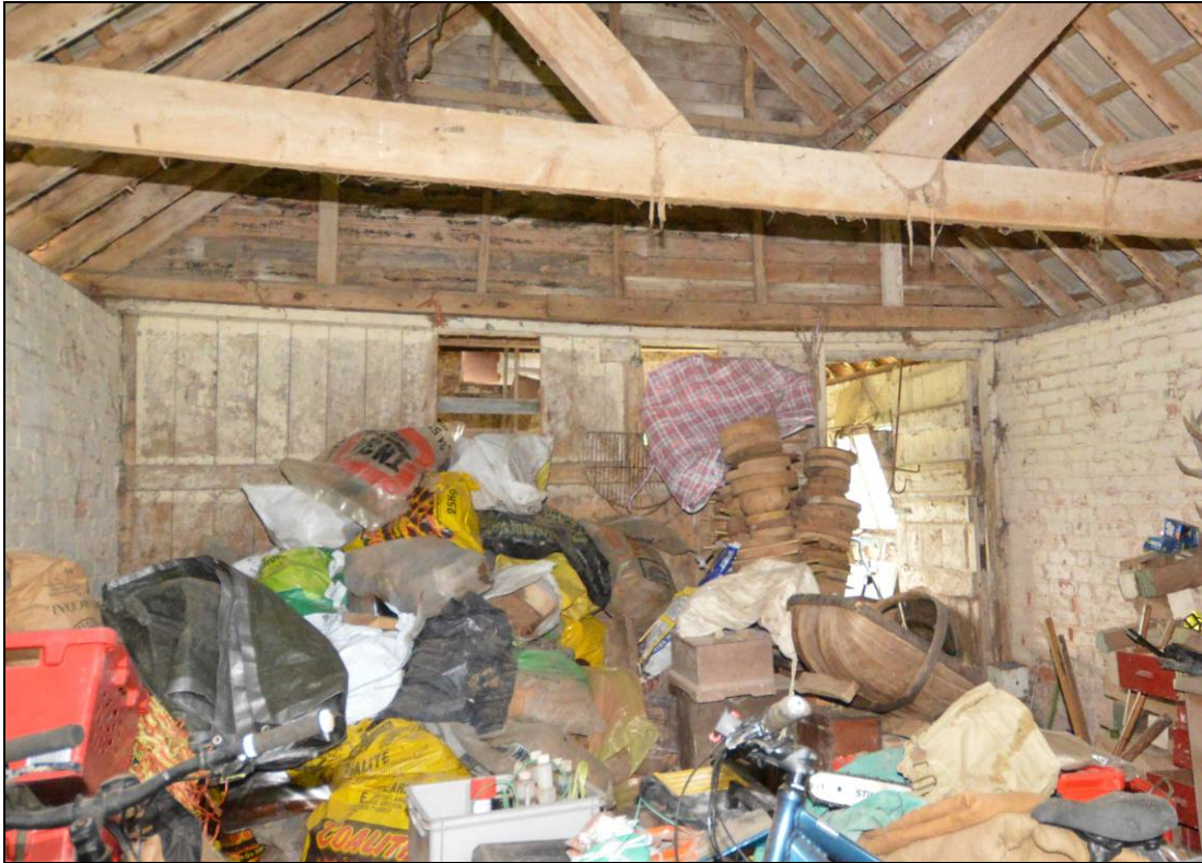
Plate 8: The light-weight timber partition separating the two rooms of the main range
