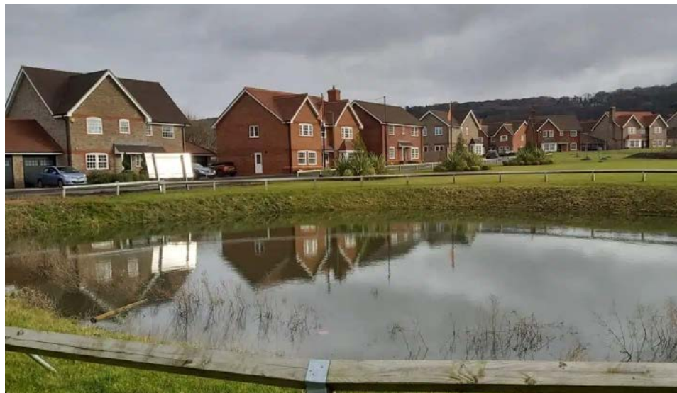
Attenuation basin to manage surface water sustainably
