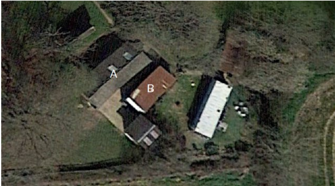
Figure 2.2 – Approved Class Q Building (A) and Structure (B) Approved for Demolition/Removal
