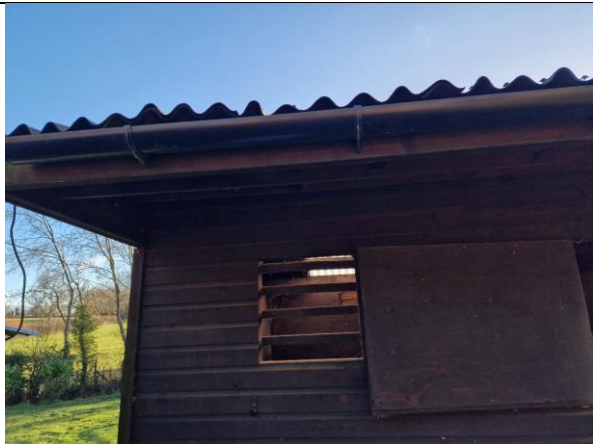
Building 3. View of building looking south east from the site.
