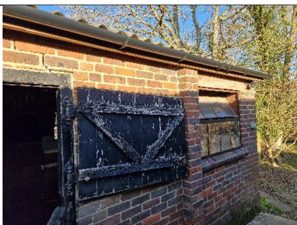
Front north view of Building 1.
