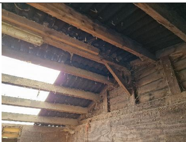
Internal view of Building 3.
