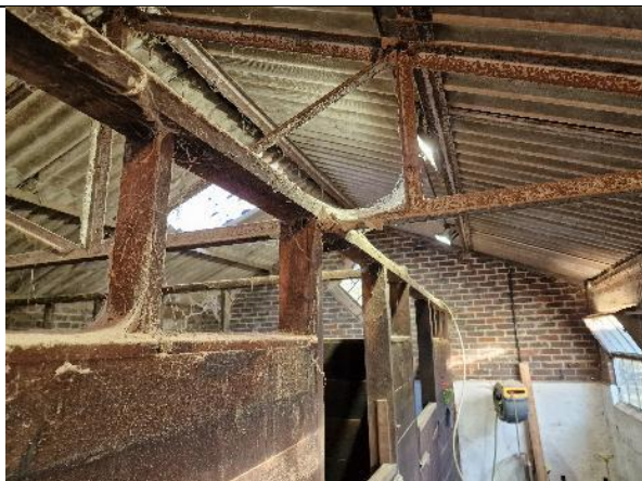
Internal view of Building 1.
