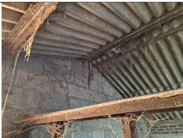
Internal view of Building 1.
