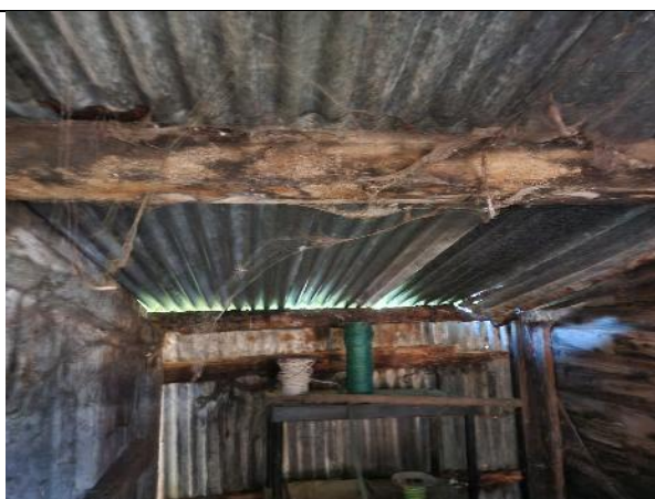
Internal view of Building 2.
