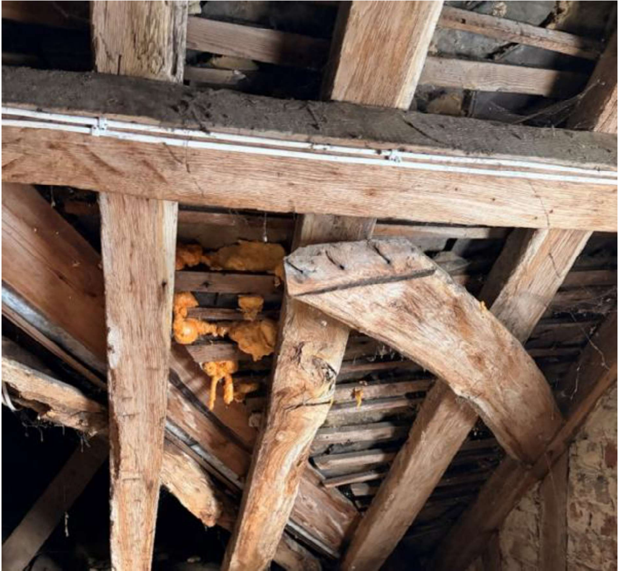
REATTACH ELBOW TIMBER
