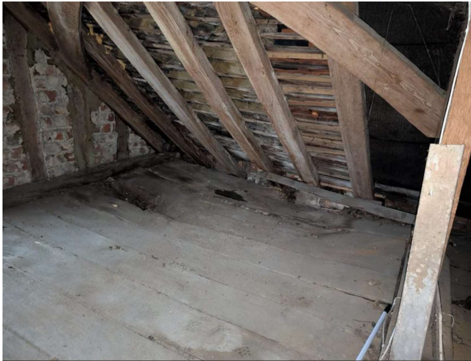
SOUTH FACING RAFTERS AND TRIMMER
