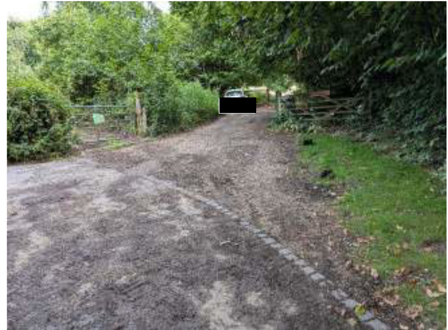
Northern access at end of works
