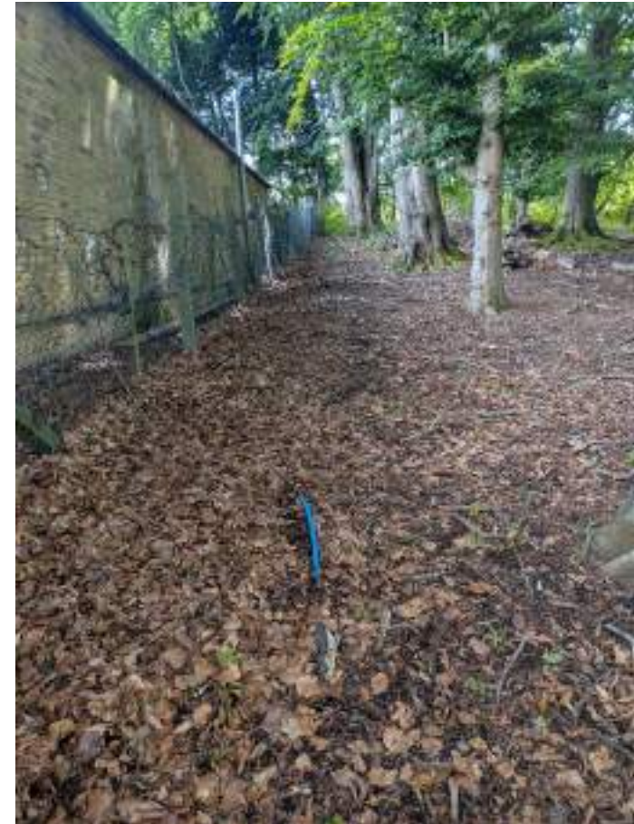
North eastern boundary of Site. Partially buried water pipeline
