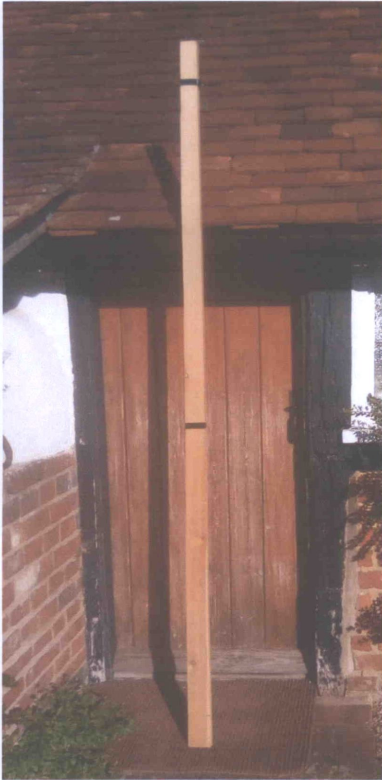
Photograph of existing back door with measuring rod marked in metres
