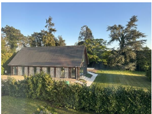
Dwelling formed from a conversion immediately to the west
