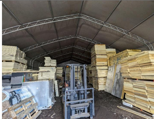
Photograph 5: Interior of the temporary structure
