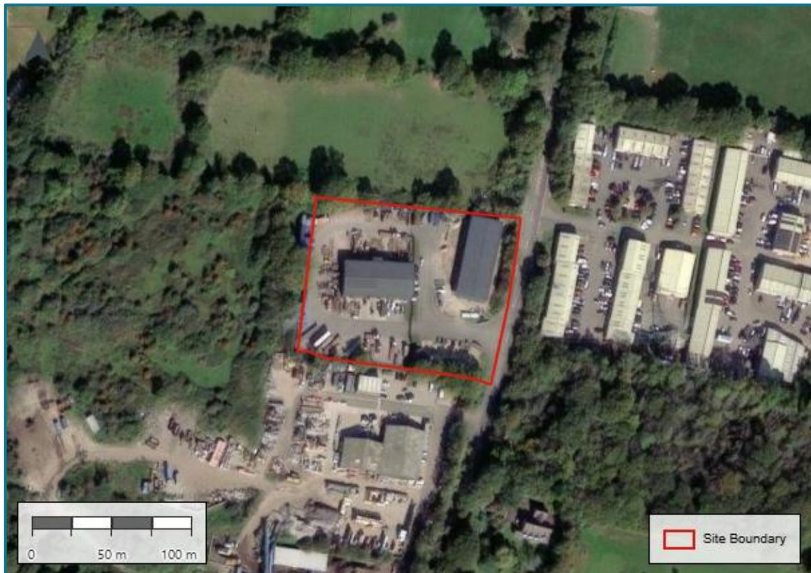
Figure 2.1 – Aerial View of Existing Site
